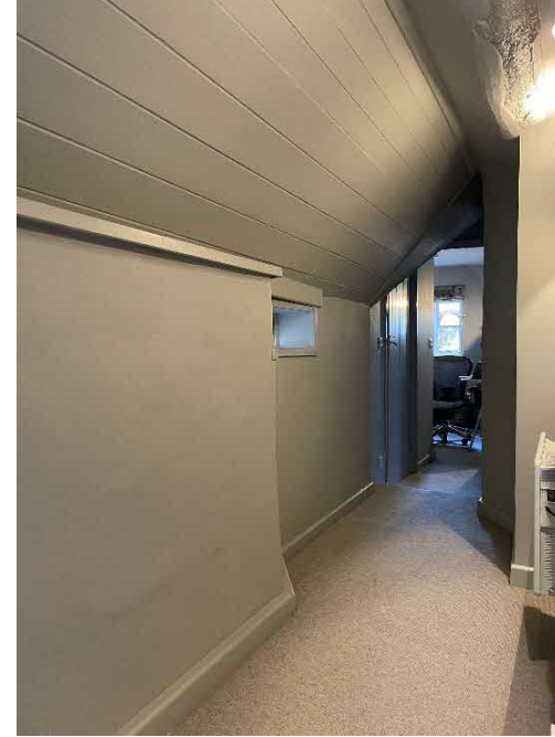
Fig 31 (bottom left) opening in central spine wall appears historic with modern plank door infill, Fig 32 (bottom centre) widened landing area and small opening in N wall, Fig 33 (bottom right) oddly pronounced purlin detail suggesting previous historic rafters removed to increase headroom above staircase.
