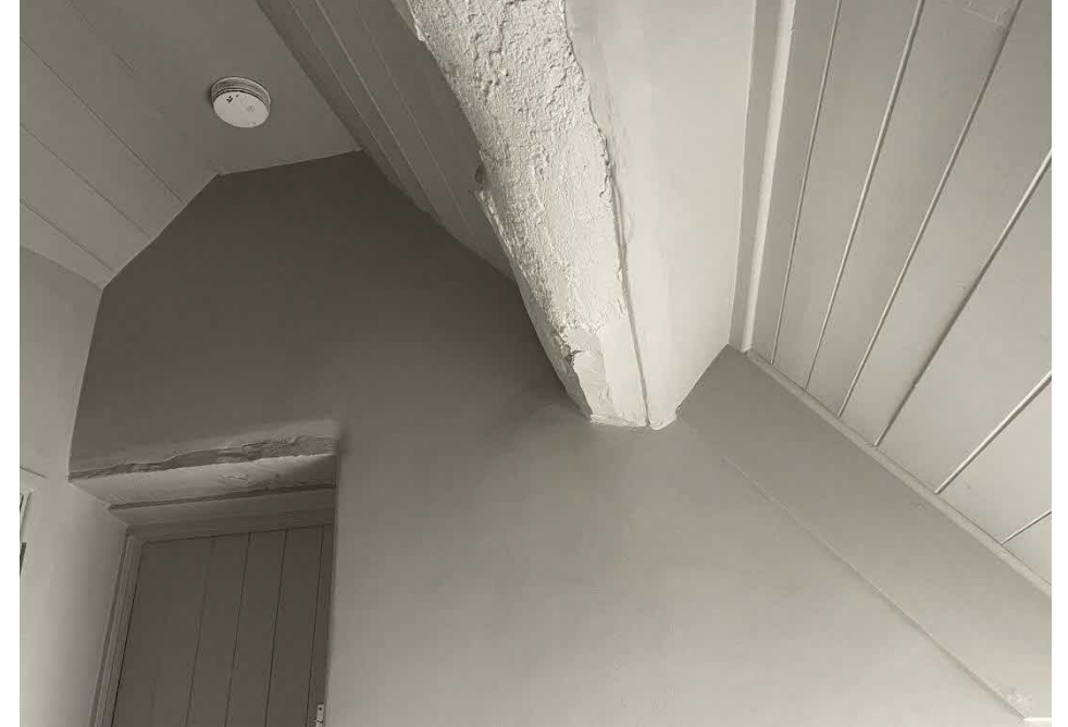
Fig 31 (bottom left) opening in central spine wall appears historic with modern plank door infill, Fig 32 (bottom centre) widened landing area and small opening in N wall, Fig 33 (bottom right) oddly pronounced purlin detail suggesting previous historic rafters removed to increase headroom above staircase.
