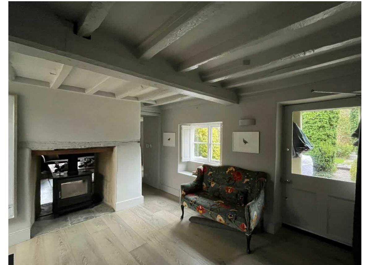
Fig 26 (top left) ground floor parlour from SE corner showing location of staircase pre 1990 (see archive images and note the two newer joists adjoining the stairs bulkhead), Fig 27 (top right) angled cuts to joist ends in NW corner of original cottage, Fig 28 (bottom left) beam detail showing the simple stops, Fig 29 (bottom right) ground floor 'parlour' with historic beam and joists and modernised fireplace.
