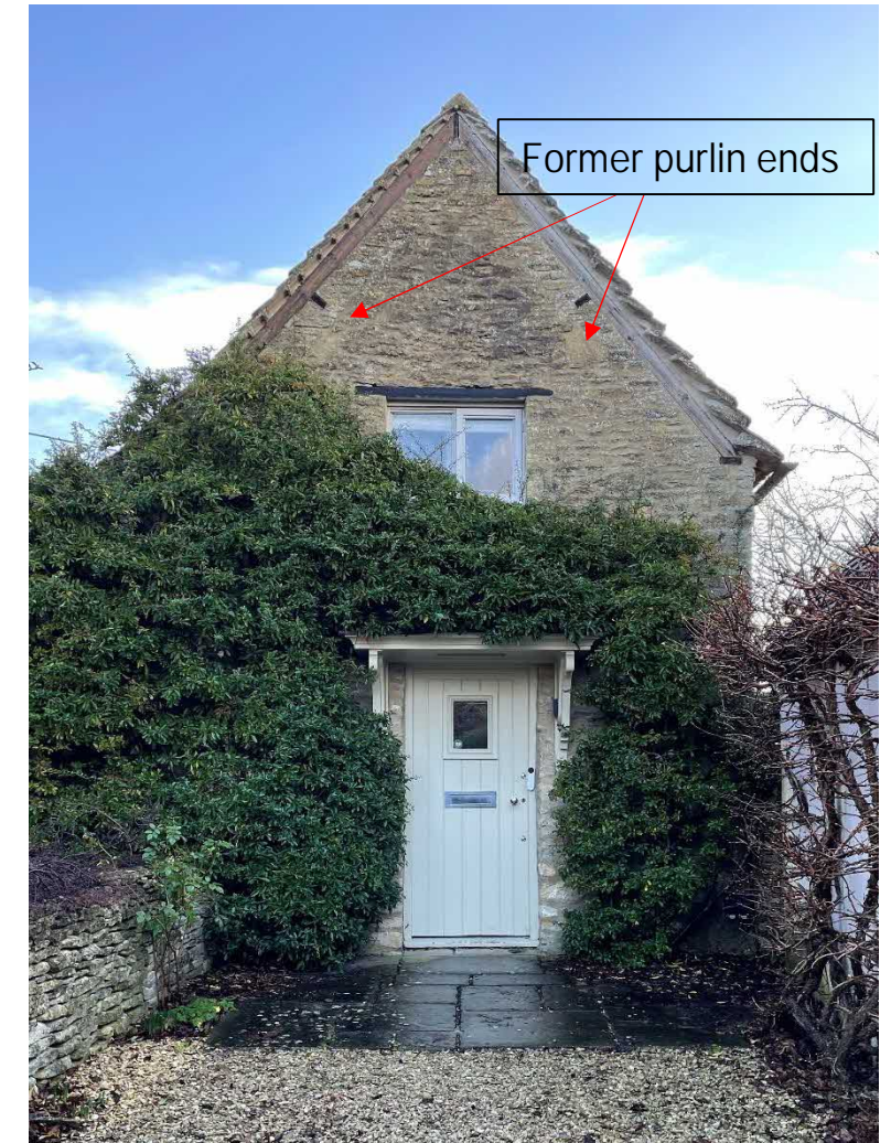
Fig 23 (top) west gable with former location of purlin ends indicated, Fig 24 (bottom left) west gable, Fig 25 (bottom right) the accumulation of modern additions to the rear northern elevation.
