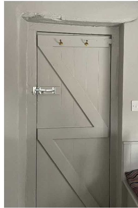
Fig 31 (bottom left) opening in central spine wall appears historic with modern plank door infill, Fig 32 (bottom centre) widened landing area and small opening in N wall, Fig 33 (bottom right) oddly pronounced purlin detail suggesting previous historic rafters removed to increase headroom above staircase.
