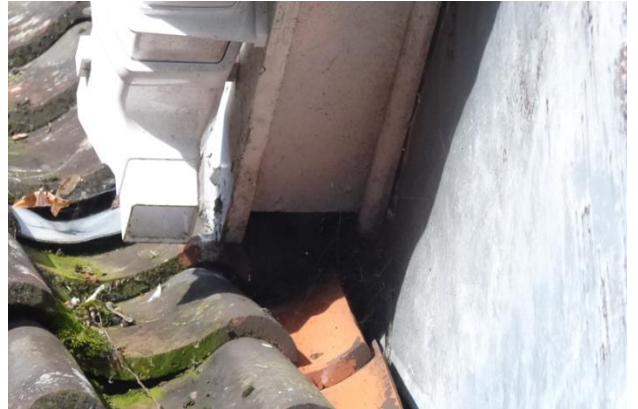
Close up view of gap
