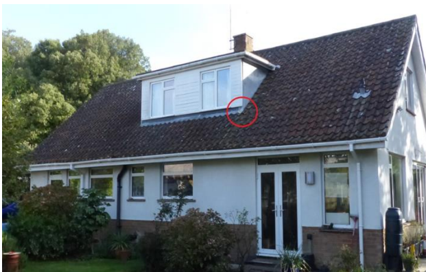
Tile gaps by dormer
