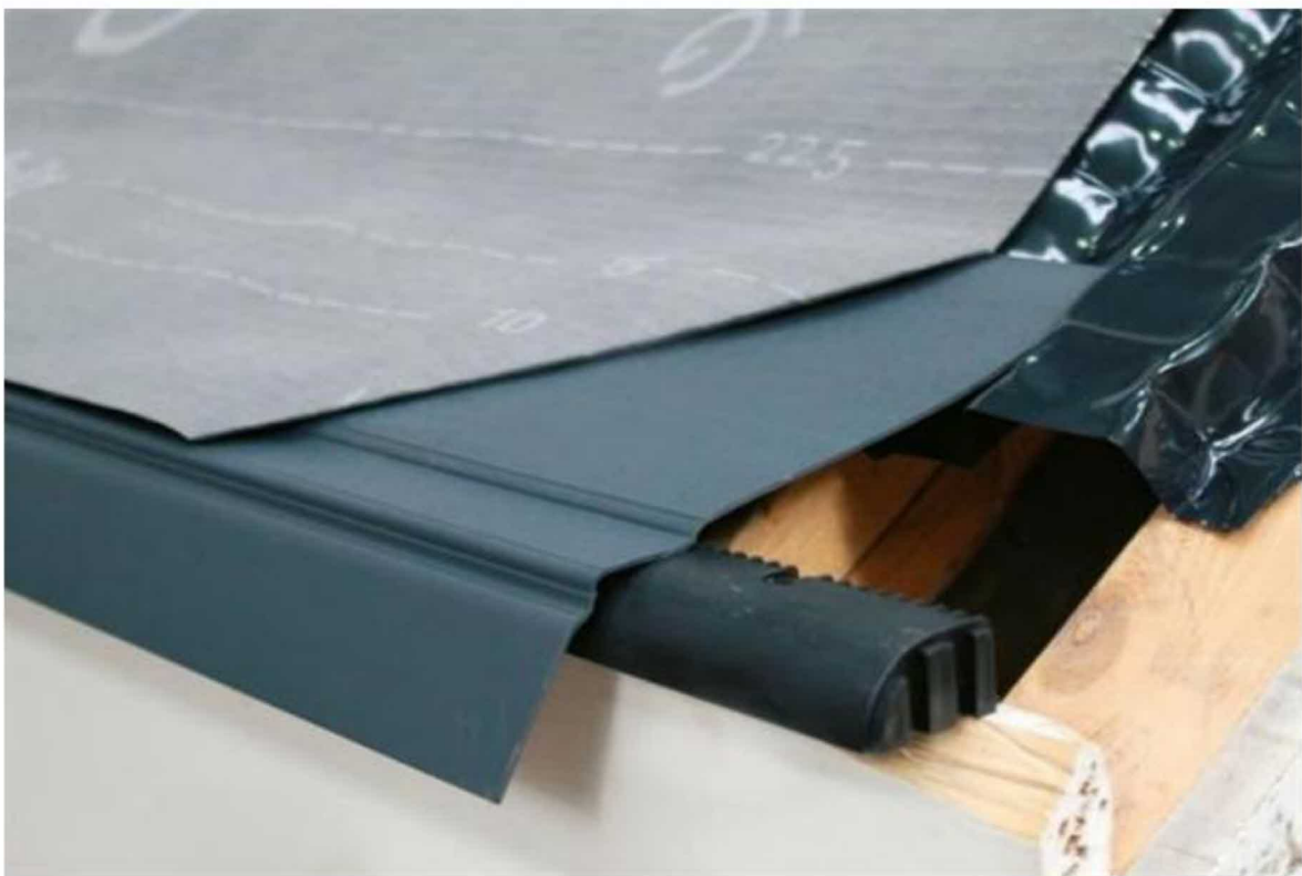
Figure 5 Extending Roofing Felt
