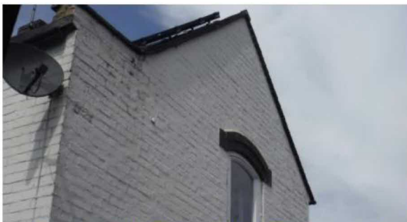
Figure 18 Gable end with flat parapet roof section
