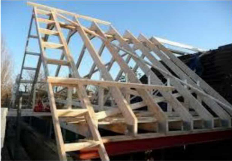
Figure 15 New build roof structure
