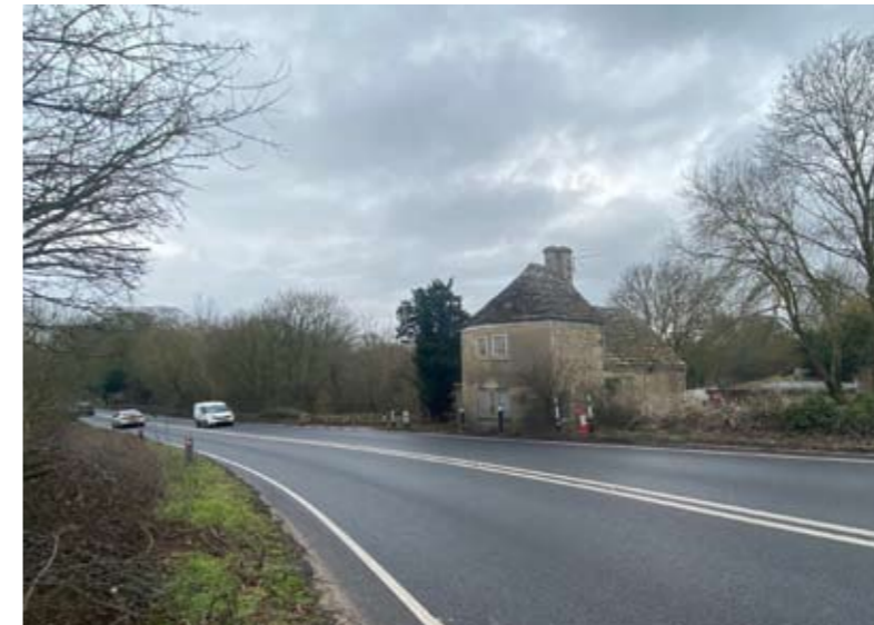
View of Tollgate Cottage looking South along A36
