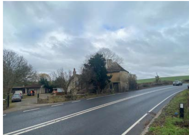
View of Tollgate Cottage looking North along A36
