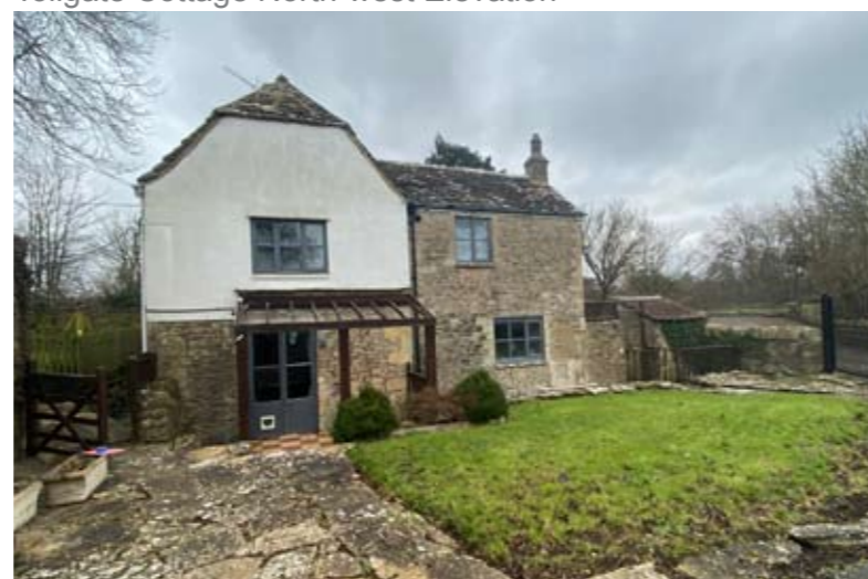
Tollgate Cottage South-west Rear Elevation
