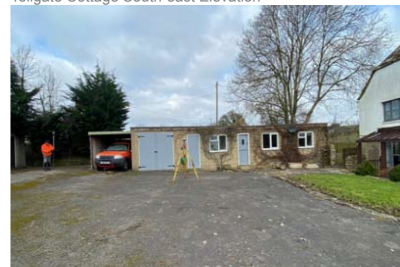
Tollgate Cottage Looking North-west toward existing Annex
