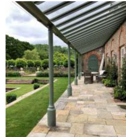
Proposed design of new painted metal verandah - Whitworth Following the simple Early Victorian column design by George Whitworth; Similar to or using this profile by the Traditional Verandah Company.
