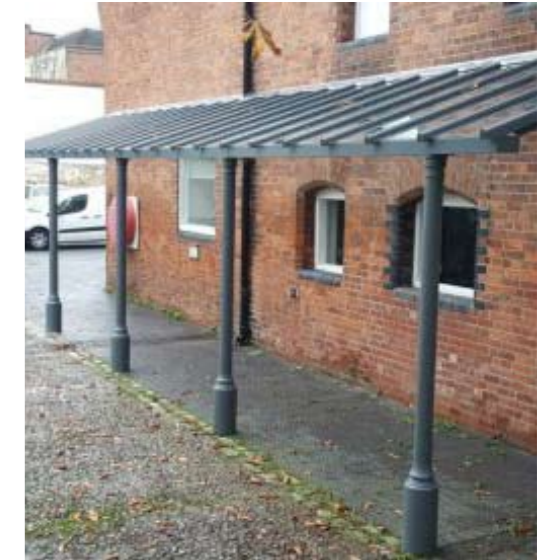
Proposed design of new painted metal verandah - Whitworth Following the simple Early Victorian column design by George Whitworth; Similar to or using this profile by the Traditional Verandah Company.
