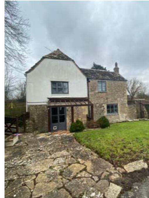
South-west view of cottage showing the existing verandah with bridges over the stream
