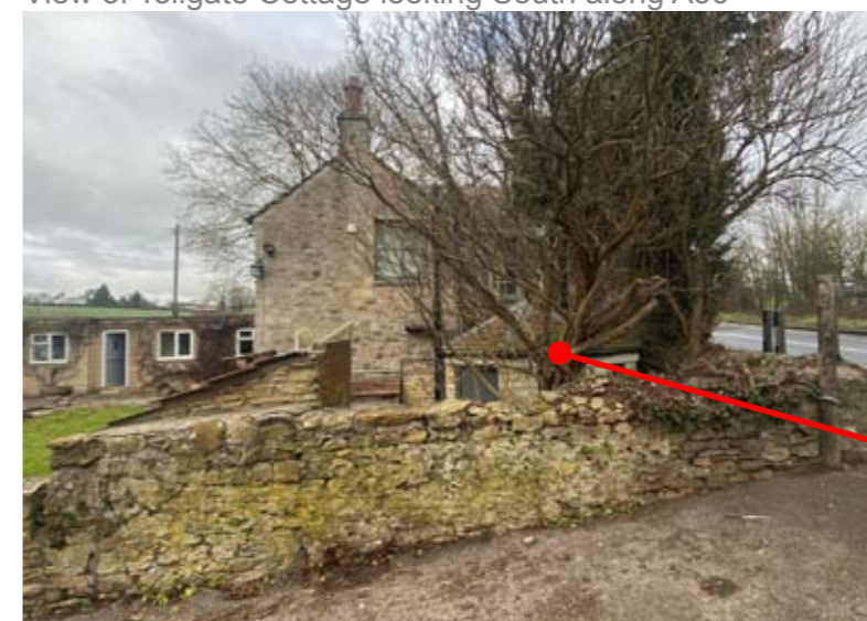
Tollgate Cottage South-east Elevation
