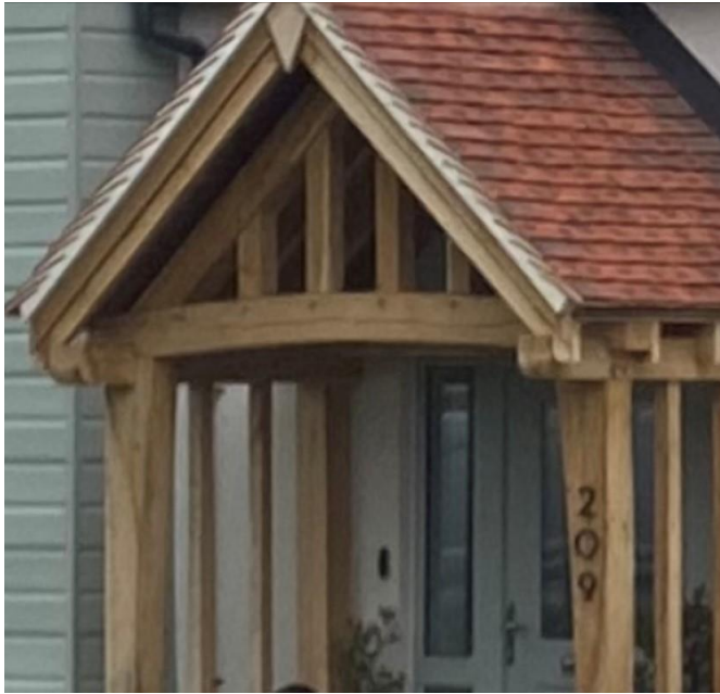
Oak framed porch posts and roof framing
