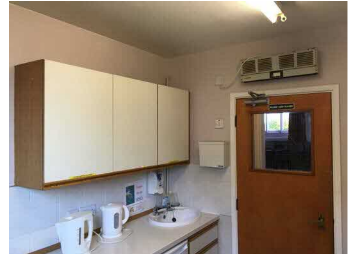
Existing kitchen - wall with door to be replaced.
