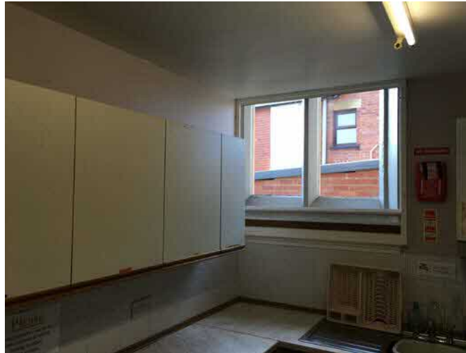
Existing kitchen - wall to left to be removed.
