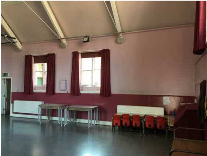
Existing hall - showing windows to be partially blocked and area of wall for new door (behind radiator).
