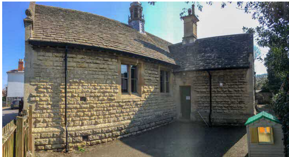
Area to be extended into - showing two windows to be partially blocked and area of wall for new opening to hall (to left of windows).
