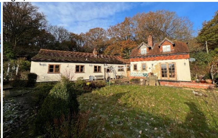
Rumplestiltskin Cottage rear from SE
