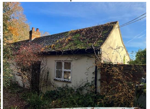
West structure SW corner
