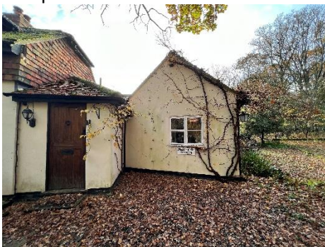
Porch & west structure N façade
