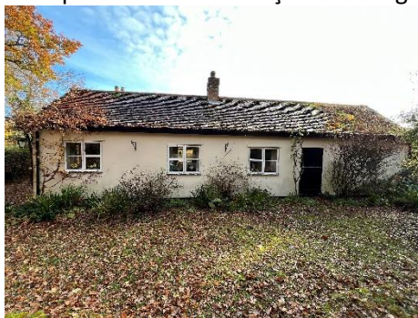
West structure west façade
