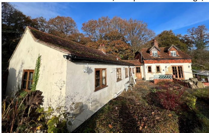
West structure S façade, roof & east structure from SW
