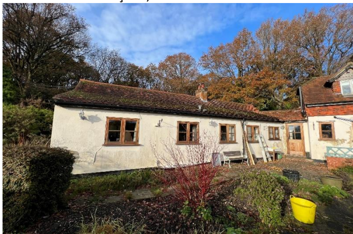
West structure & porch from south east
