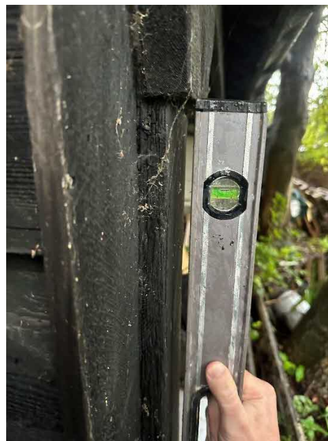
Fig 1.3 Movement to the rear wall and Timber Post structure
