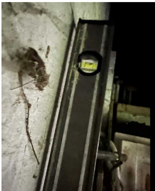
Fig 1.3 Movement to the rear wall and Timber Post structure
