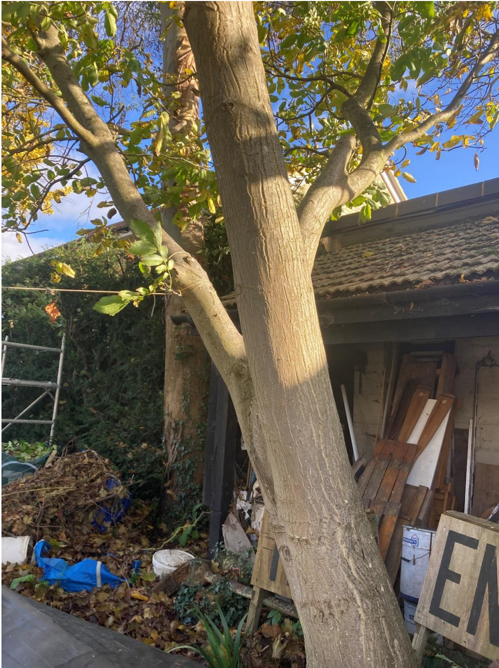
Photograph 6 Proximity of trees to outbuilding and lean on walnut
