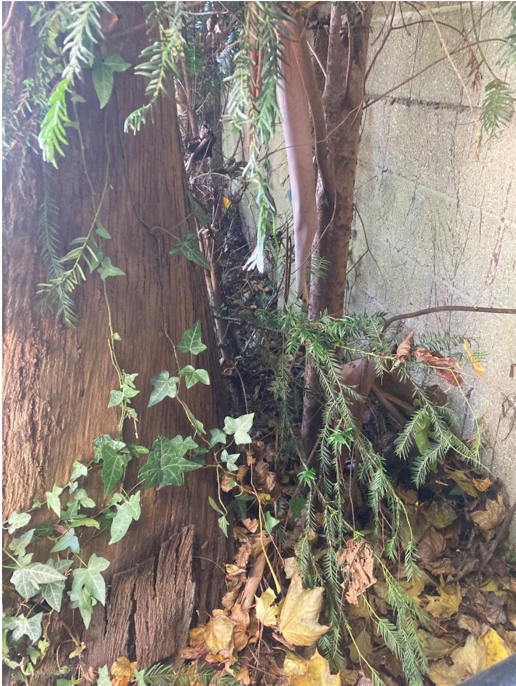
Photograph 5 Proximity of party wall
