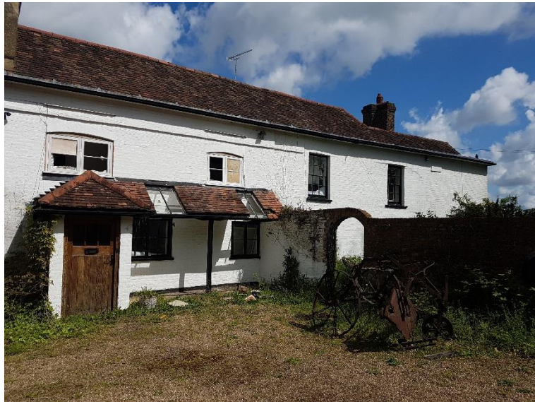
Fig 7. View of the Farmhosue looking north within the site.
