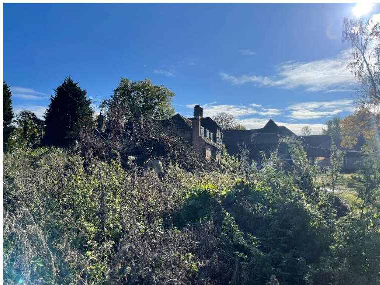
Fig 11. View of the Farmhouse and Barn looking west within the site.
