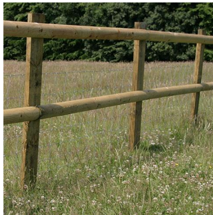
Fig 42. Proposed post and rail timber fence.
