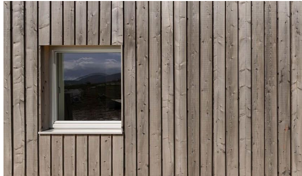
Fig 33. Untreated Scottish larch vertical cladding
