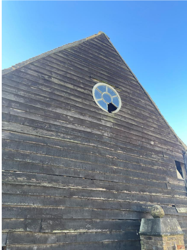
Fig 20. Existing circular window and timber cladding to the Barn
