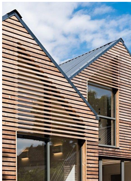
Fig 28. Example of hit and miss timber cladding over windows
