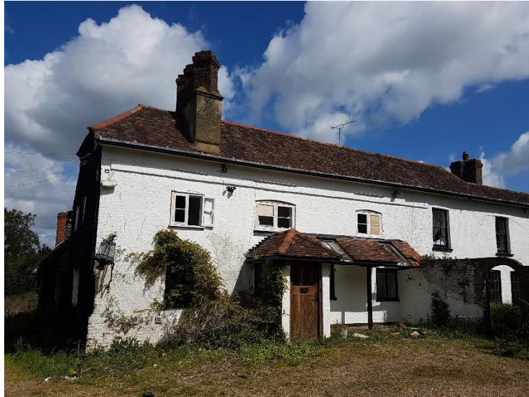
Fig 6. White washed wallss to existing Farmhouse
