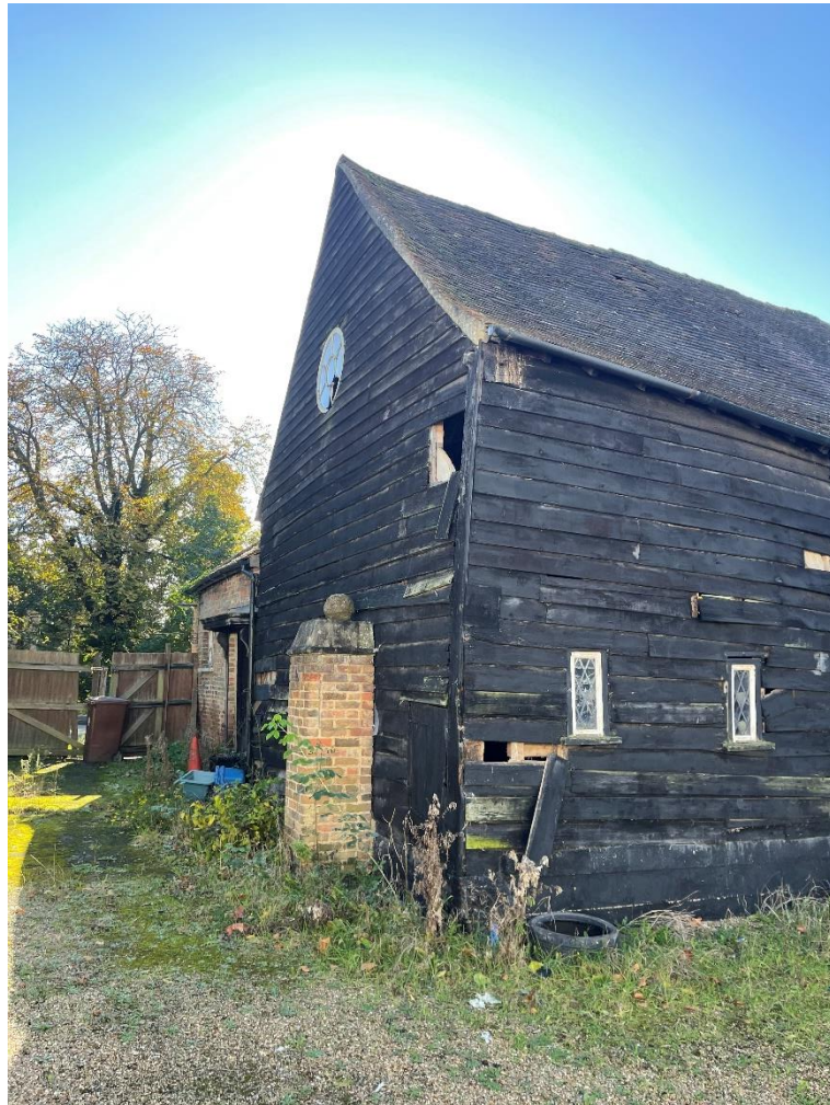
Fig 19. View looking south at the existing Barn with gated access to Allum Lane
