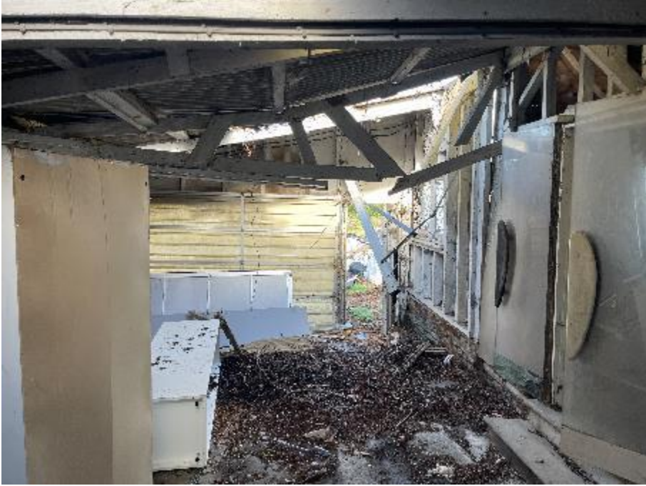
47. Garage 'K' looking north
