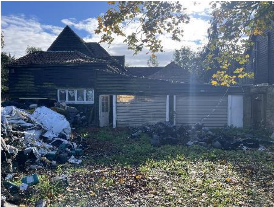
16. Barn garage to north
