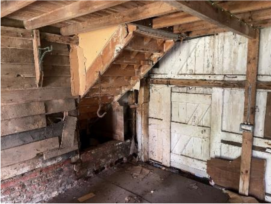
43. Room 'H' looking west
