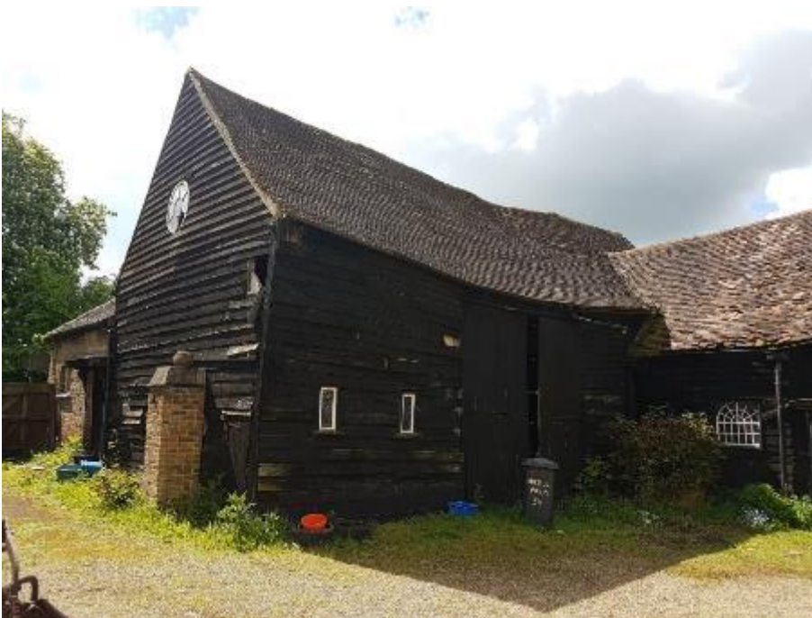
12. Barn from north-east
