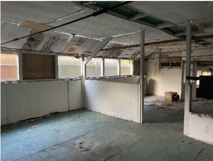
48. Room 'L' looking west
