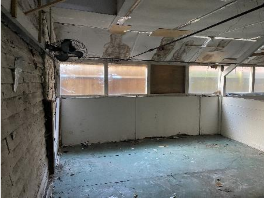
49. Room 'L' looking west
