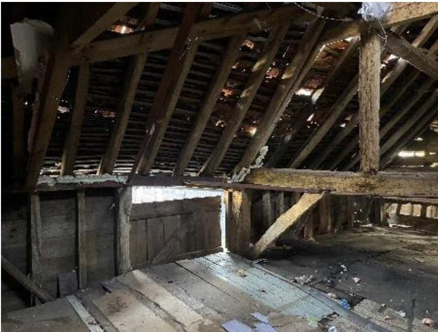
54. Room 'P' looking east
