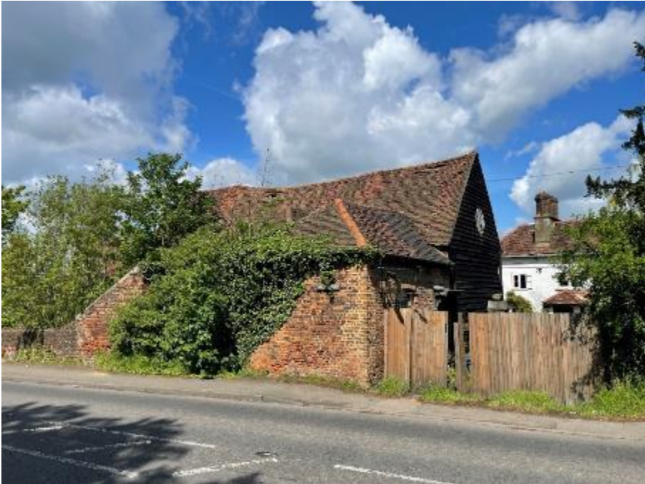
1. Barn from south-east
