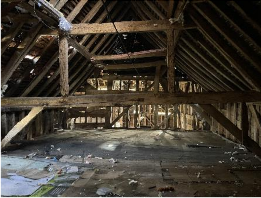
53. Room 'P' looking south
