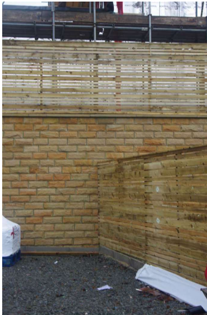
Stone walling to plot retaining wall
