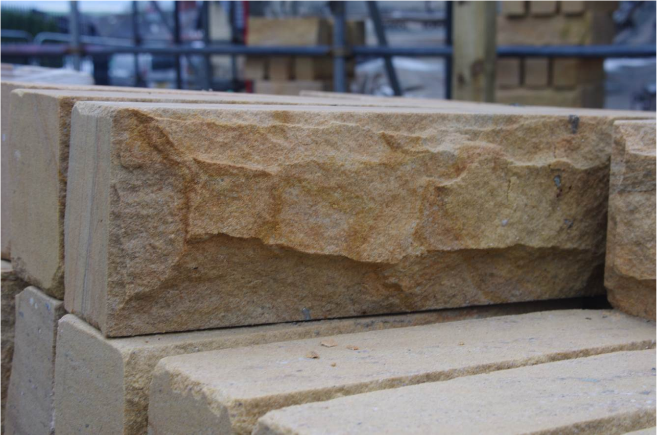
Typical natural 'split face' stone walling
