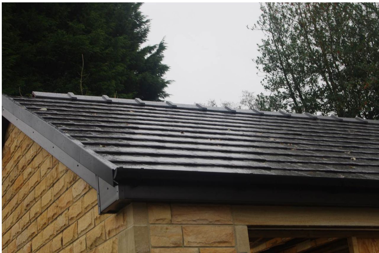
Typical view of garage walls & roof
