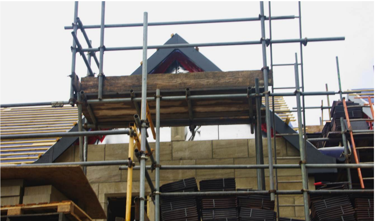
Ashlar panel to front elevations
