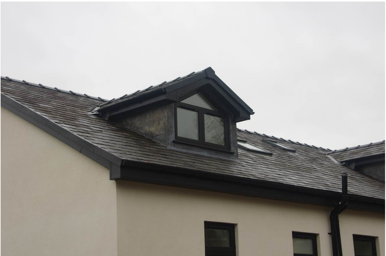
Typical rear view of render walls, slate roof & lead dormers
