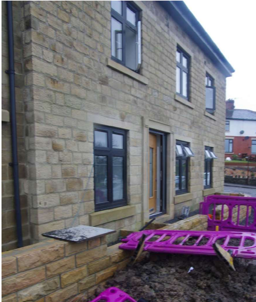
Rebuilt front elevation to Plot 1
