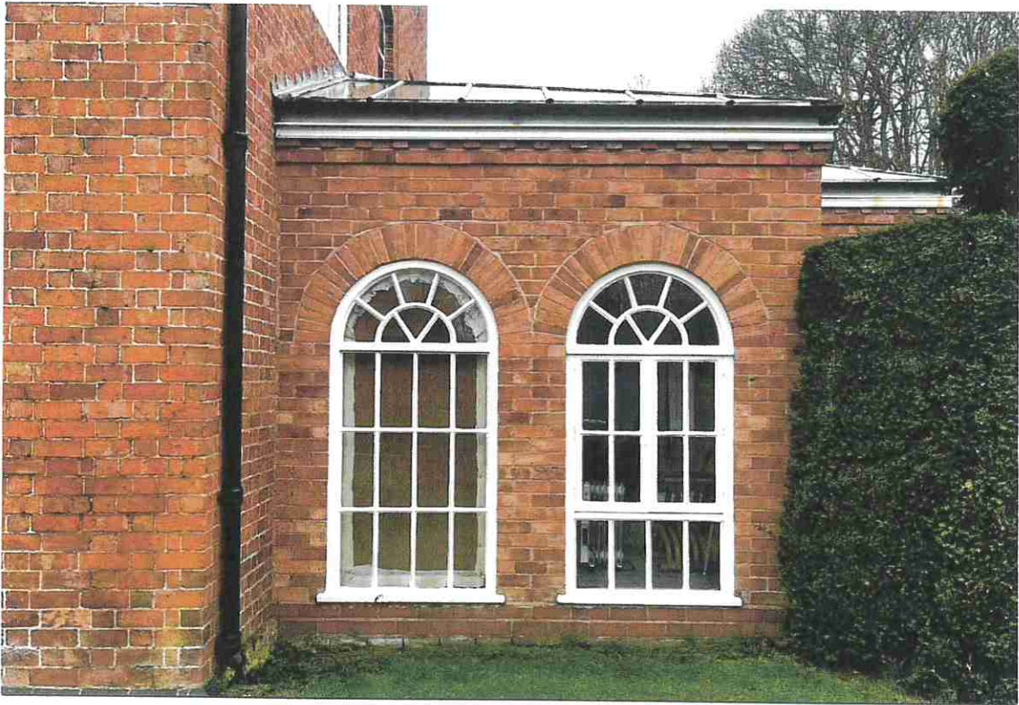
PHOTOGRAPH 4 - DETAIL OF NORTH WEST ELEVATION OF THE EXISTING GARDEN ROOM.
