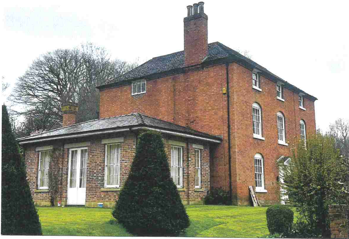
PHOTOGRAPH 12 - GENERAL VIEW OF THE SINGLE STOREY DINING ROOM EXTENSION ON THE NORTH EAST SIDE OF THE HOUSE WHICH HAS A NATURAL SLATE ROOF FINISH.
