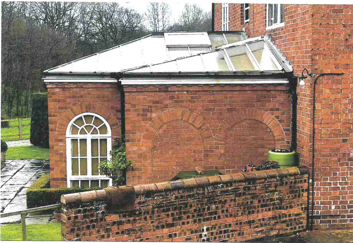
PHOTOGRAPH 5 - DETAIL OF THE SOUTH EAST ELEVATION OF THE EXISTING GARDEN ROOM.
