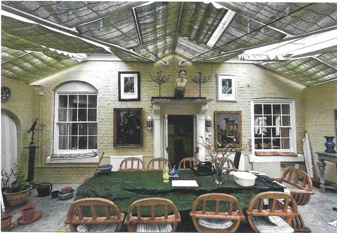
PHOTOGRAPH 8 - GENERAL VIEW OF THE INTERIOR OF OF THE EXISTING GARDEN ROOM LOOKING BACK TOWARDS THE ORIGINAL HOUSE.
