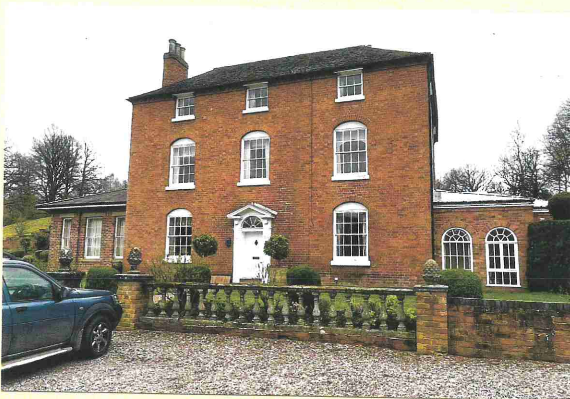
PHOTOGRAPH 1 - GENERAL VIEW OF SHEINWOOD MANOR, WITH THE EXISTING GARDEN ROOM ON THE RIGHT.
