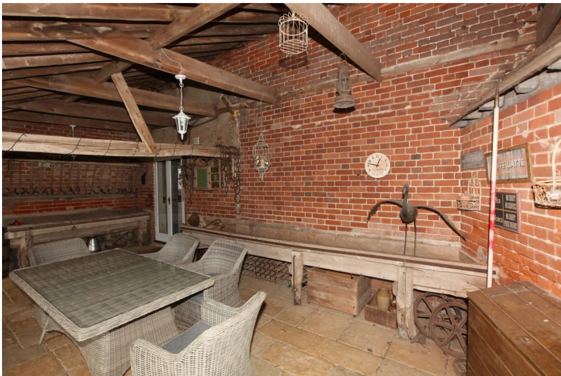
Illus. 34. The 19 th century boarded manger against the northern internal wall of the shelter-shed in the cow yard (3) with the modern French doors to the house on the left. This manger is understood to have been moved from the horse yard's shelter-shed to the south of the outbuilding (1).
