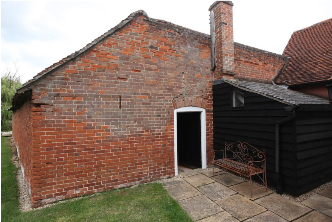
Illus. 11. The northern gable of the outbuilding which is integral to the wall of the cow-yard's shelter-shed (3) on the right and effectively screens the farm yard from the house. The arched doorway is also integral to the Flemish Bond brickwork and opens directly into the compartment described in 1938 as a mixing house (2a).
