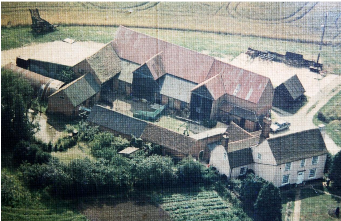
Figure 15 Aerial photographs probably from the 1970s and 90s in the current owners' possession. The southern threshing barn retains its original thatch in the former while the later image below shows corrugated iron on both the barn and the southern half of the outbuilding in the foreground. The walls of the small cattle yard to the north of the outbuilding still survived in the 1970s but had been lost by the 1990s.
