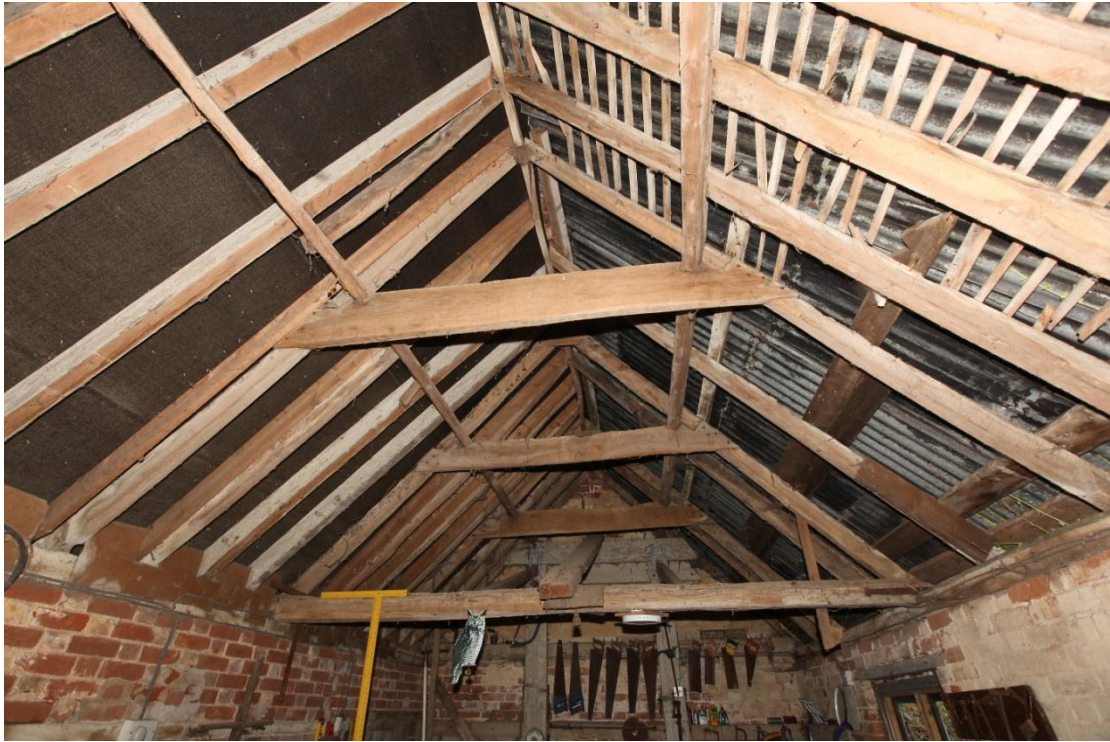
Illus. 19. The partly intact original clasped-purlin roof structure of the cow shed (2) as seen from the north. The rafters rest on a ridge-board and the original collars are nailed rather than pegged as might be expected in a relatively narrow structure. The original tile battens survive to the right.
