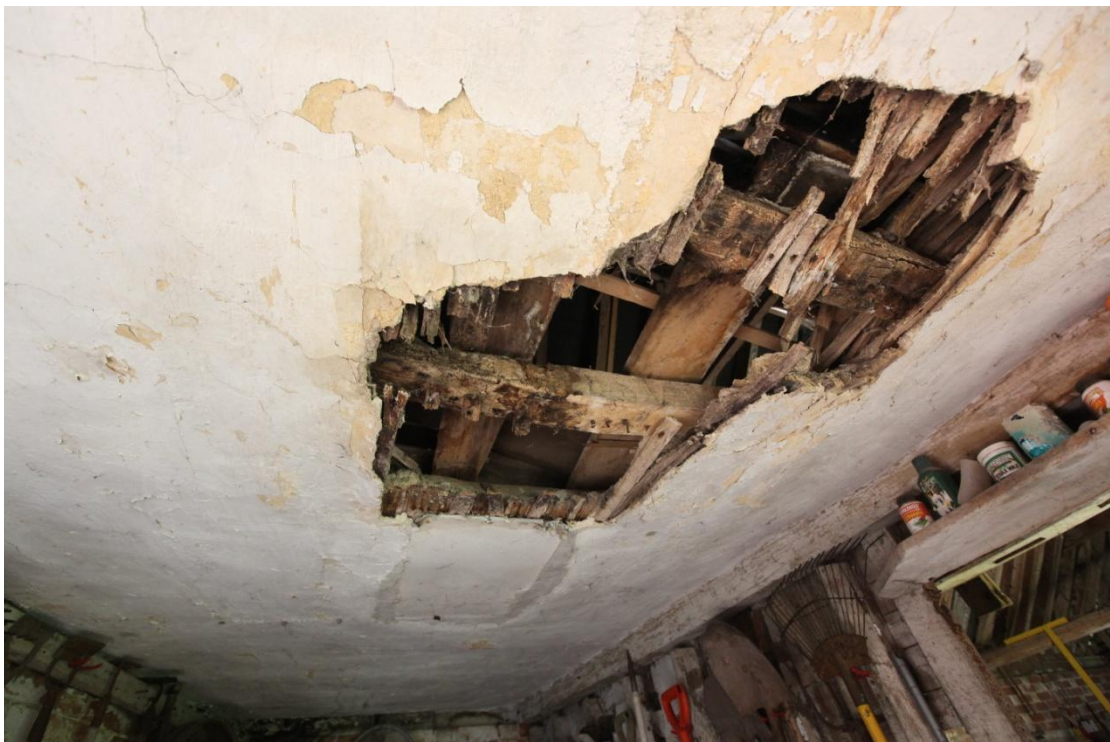
Illus. 26. A detail of the 19 th century lath-and-plaster ceiling of the mixing house (2a) as seen from the west. The laths are nailed to the undersides of the original common joists. There is no evidence of whitewash on either the joists or the upper laths in illustration 22 that might suggest this plaster post-dates the layer of clay daub above.
