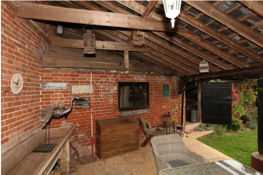
Illus. 33. The interior of the shelter-shed (1) to the north of the farm yard showing the window to the mixing house (2a) in the cow shed. This window is modern but its aperture is respected by closers in the brickwork.
