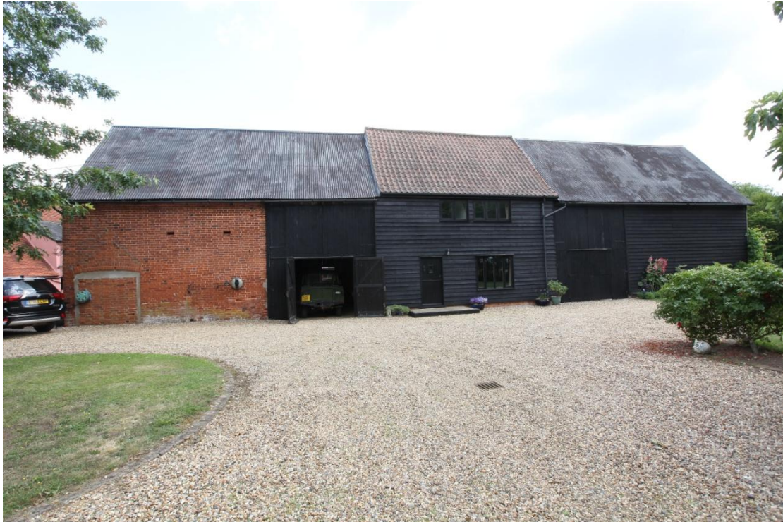
Illus. 7. The barn from the west showing the raised roof of the central section which has been converted into a dwelling (included for site context). The brick bay on the left was described as a corn barn in 1938 and contains a blocked unusual arched entrance to the extreme left. It probably operated in the manner of a modern grain store.
