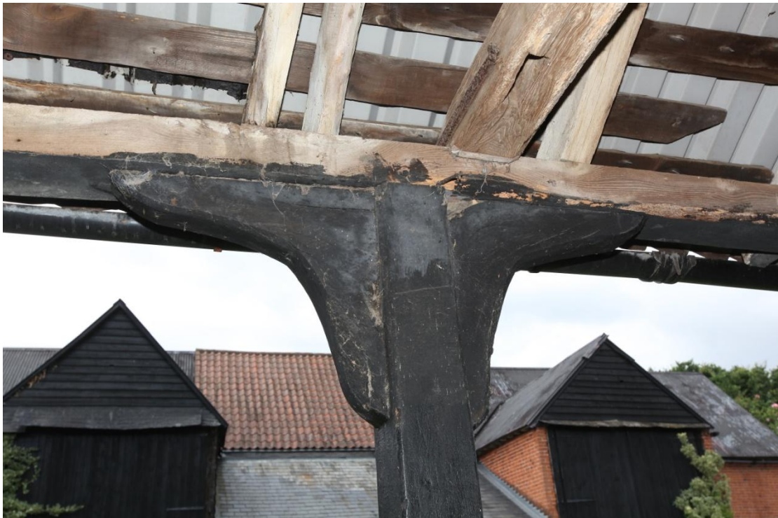
Illus. 16. A detail of the original tarred and bolted knee-braces linking the arcade post of the horse shelter-shed's western interior to its roof-plate (1).
