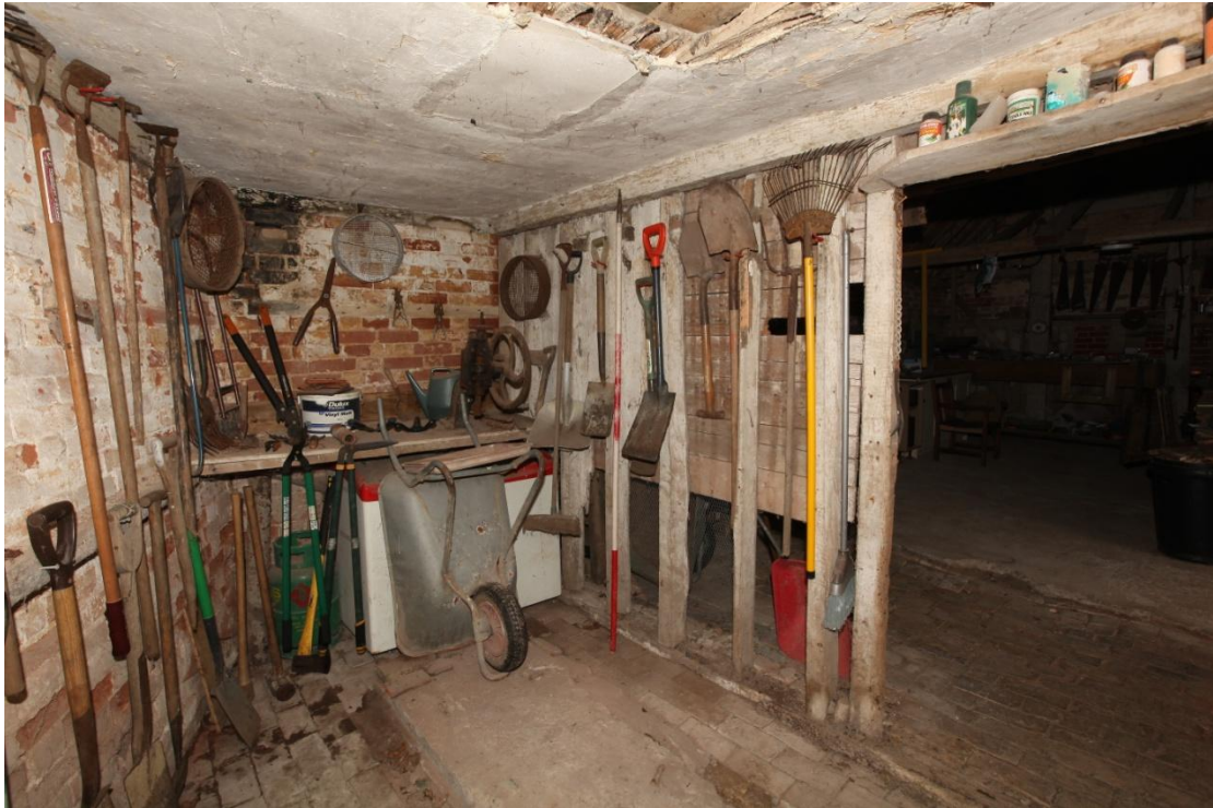
Illus. 25. The interior from the west of the mixing house (2a) showing the brick northern gable on the left and the entrance to the main cow shed (2) on the right. The mixing house varies from 1.4 m in length against the eastern wall in the centre to 3 m on the west, reflecting the irregular angle of the building's corner.
