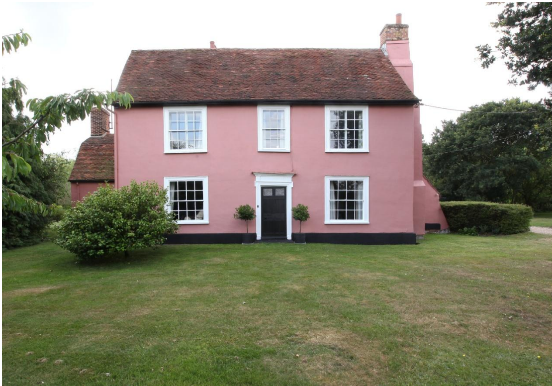
Illus. 1. The northern facade of the former farmhouse, which faces the road and conceals the farm yard to the rear. Listed as 18 th century, the internally exposed framing consists of narrow studs interrupted by straight primary braces which are pegged rather than nailed at each end in the manner of the late-18 th and early-19 th centuries.
