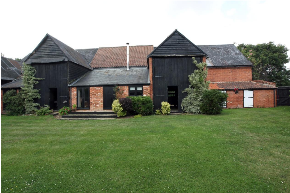
Illus. 5. The double threshing barn to the west of the yard, with lean-to loose boxes between its porches (included for site context). The brick bay on the right appears to have been built as an extension to the earlier and formerly thatched barn on the left.
