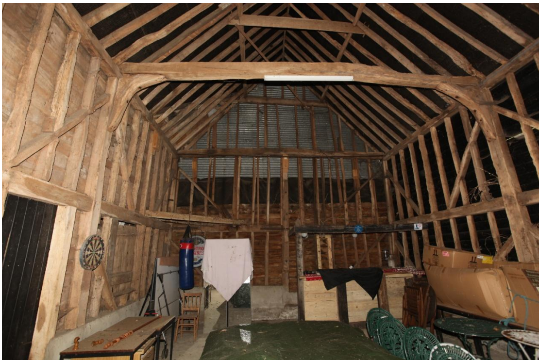
Illus. 8. The internal southern gable of the threshing barn showing its typically early-19 th century framing with original bolted knee-braces rather than arch-braces to the tie-beam (included for site context). It is stylistically slightly later than the house as its diagonal wall braces are nailed rather than pegged, although the roof collars are pegged.
