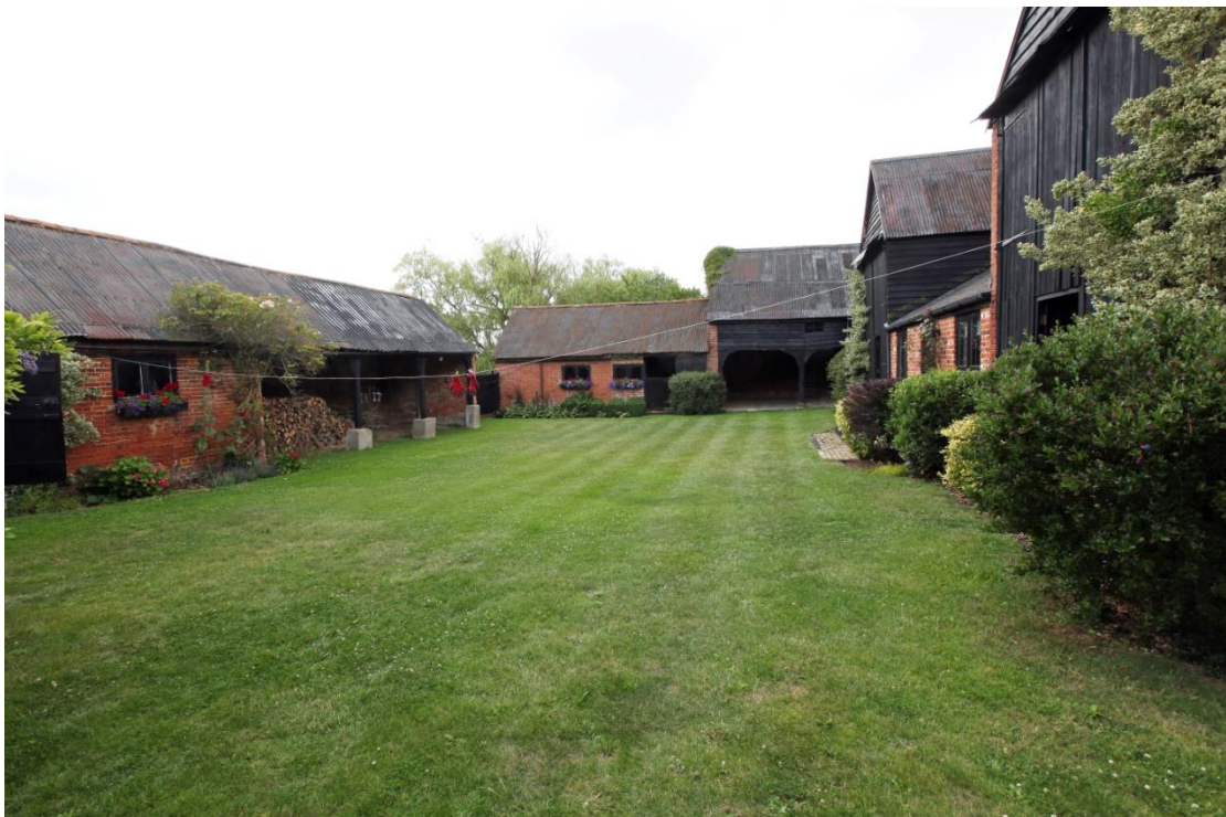
Illus. 4. The enclosed farm yard from the north showing the outbuilding on the left with the brick stable and boarded granary in the rear and the threshing barn on the right. The buildings are all consistent with the date in the 1820s or 30s indicated by the historic maps.
