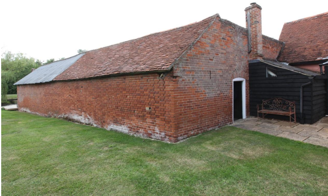
Illus. 10. The outbuilding from the north-east showing its Flemish Bond fabric with the boarded shed of the house adjoining on the right and the original entrance doorway in the northern gable of the feed-mixing shed (2a).
