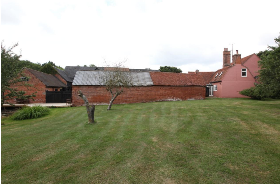
Illus. 9. The brick outbuilding from the east showing the stable on the left and the house to the right. The structurally distinct section of the house with a gambrel roof was added between 1837 and 1885 according to the historic maps. The tiles of the left-hand section of the outbuilding were replaced with corrugated iron between the 1970s and 90s as indicated on the aerial photographs in figure 15.
