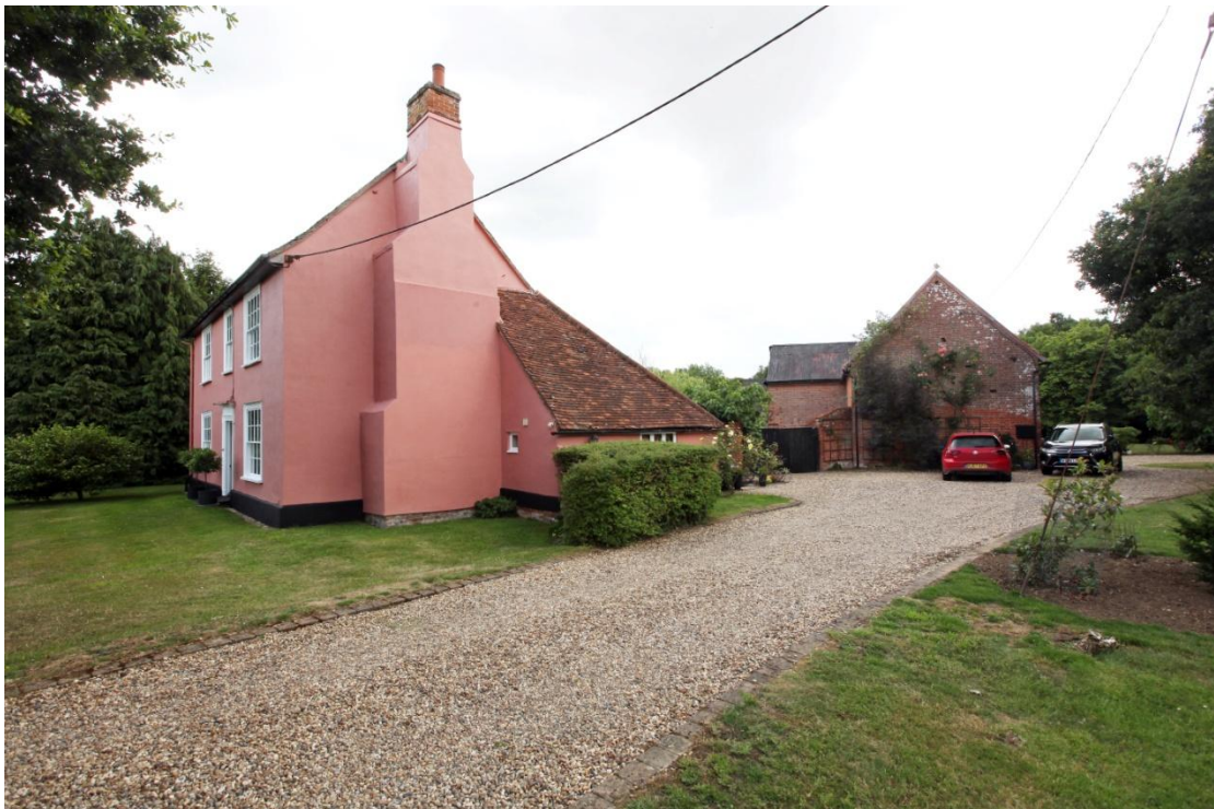
Illus. 2. The house from the entrance drive to the north-west showing the brick extension to the earlier thatched threshing barn in the rear.
