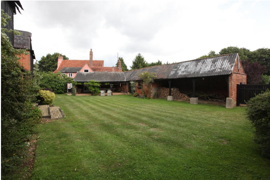
Illus. 3. The enclosed farm yard from its south-western corner showing the L-shaped outbuilding on the right with the 3-bay open shelter-shed of the horse yard (1) on the right, the cow shed (2) in the centre and the shelter-shed of the cow yard (3) on the left. The threshing barn is visible to the extreme left with the house in the rear.
