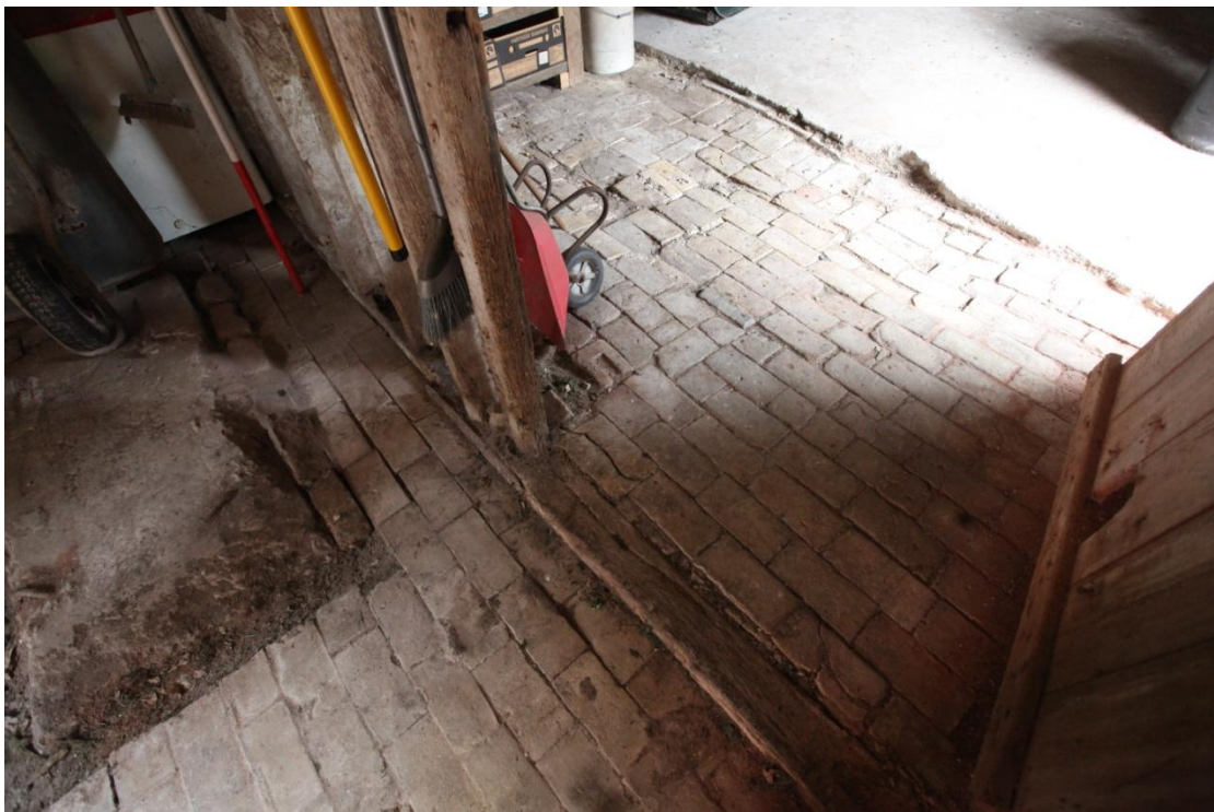
Illus. 30. The 19 th century floor bricks of the mixing house (2a) on the left and the main cow shed (2) on the right. The bricks respect the sill of the partition between these spaces, suggesting it is contemporary with the building. The concrete blocked to the left supported a missing 20 th century tank.
