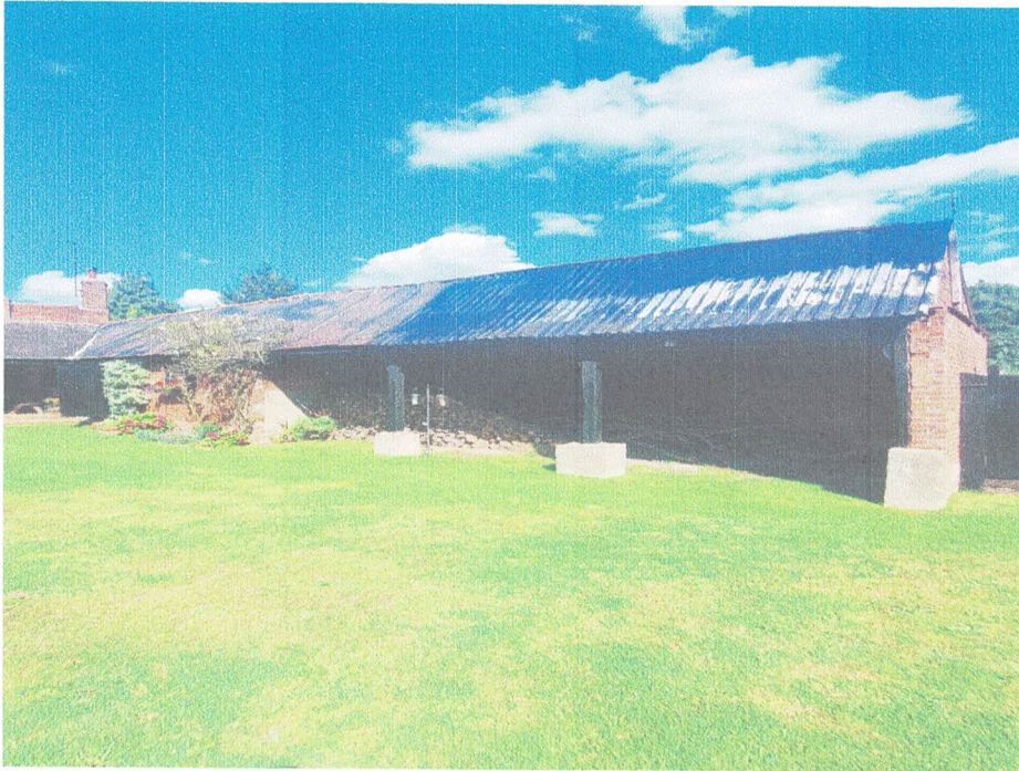
P1 – General view of front elevation to cart lodge and workshop.
