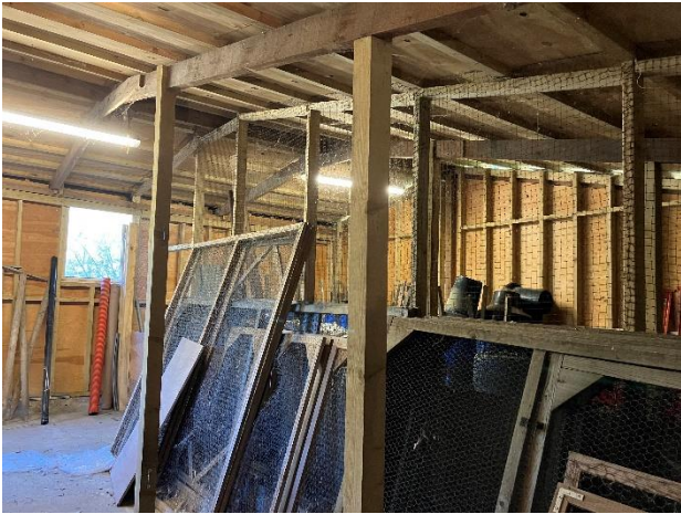
Photo 5: Internal view of main building section
