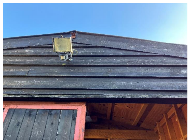
Photo 2: Closely fitting barge boards across weatherboarding, which is in good condition
