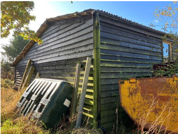
Photo 7: North eastern elevations of the building
