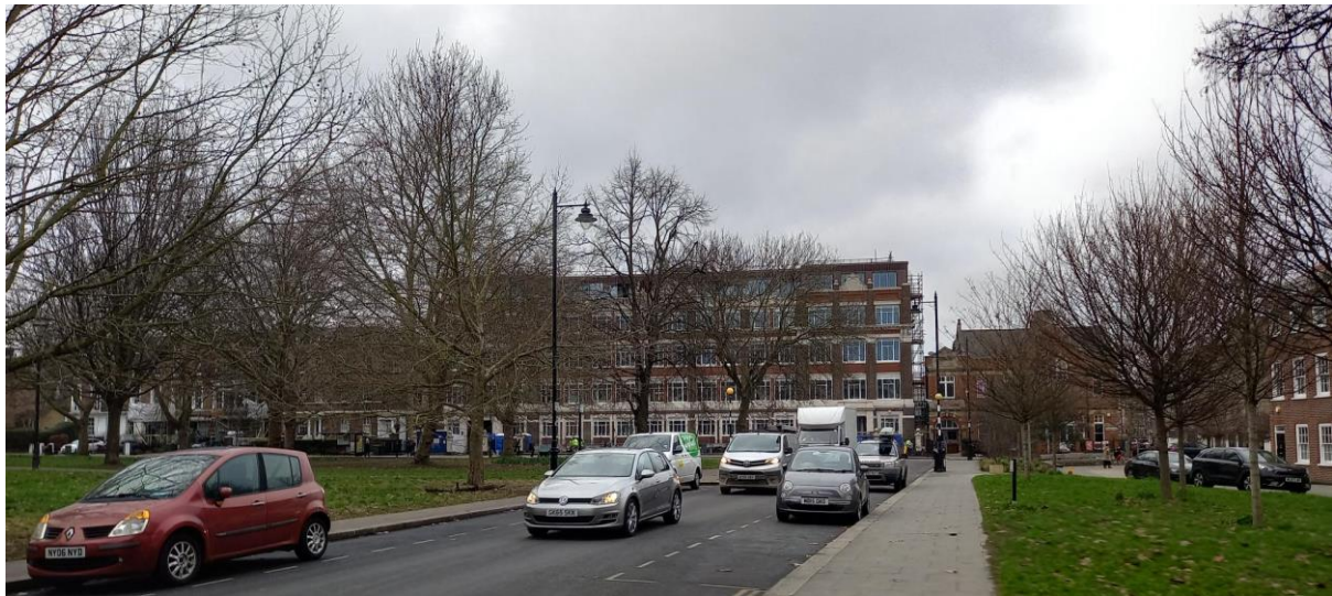
Fig7. Photo of GWH with rooftop structure from a site visit on 21/02/2023
