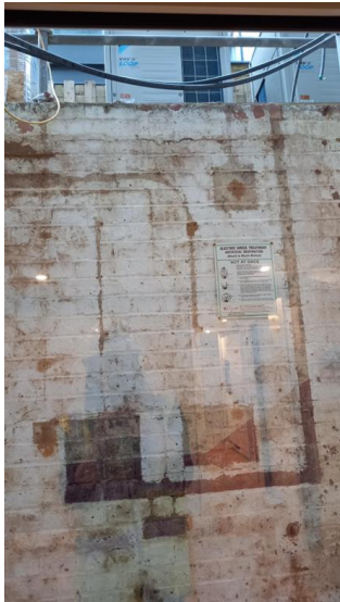
Fig5. View from basement level flat when looking from the closed rear door
