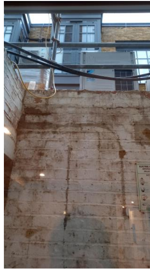
Fig6. View from outdoor terrace basement flat when looking up
