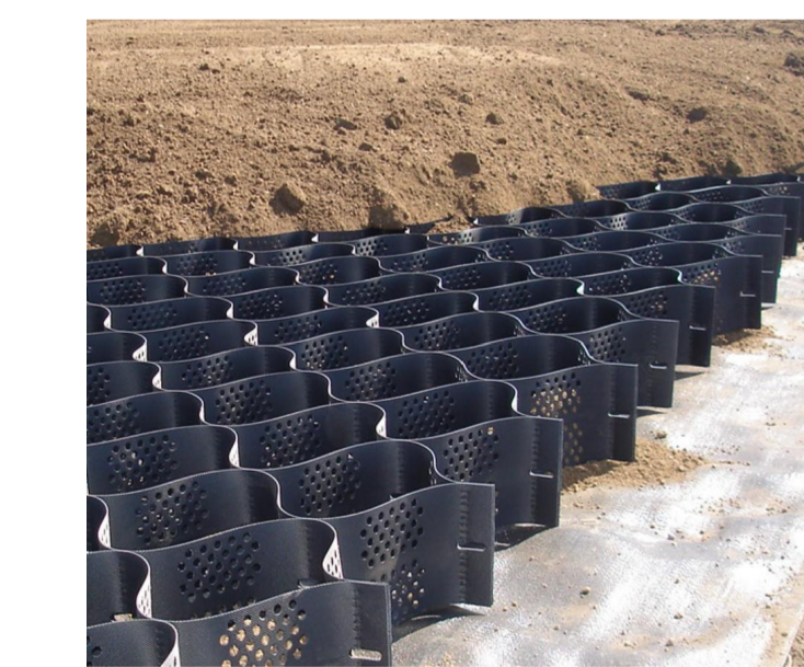
Fig.2 Cellular confinement system over permeable weed barrier sheeting. Pegged and edged to create a stable sub-base and filled with no-fines aggregate. System does not need compaction, and should minimise impact on the areas of RPA proposed as driveway.
