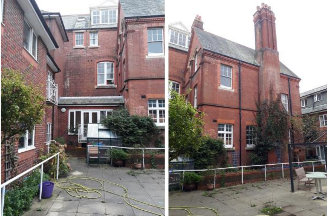
Front elevation, courtyard view
