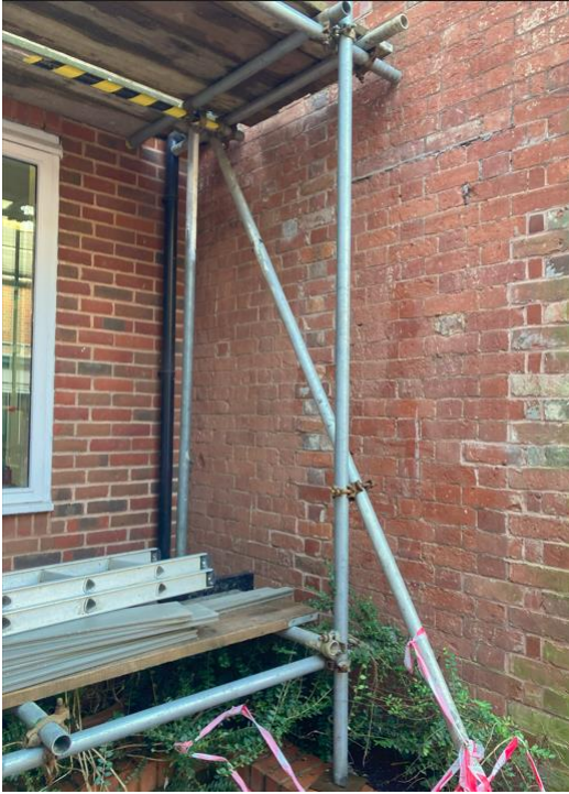
South courtyard Change in brickwork from original to new
