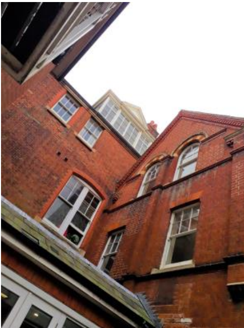
South courtyard: 1st floor of southern recess
