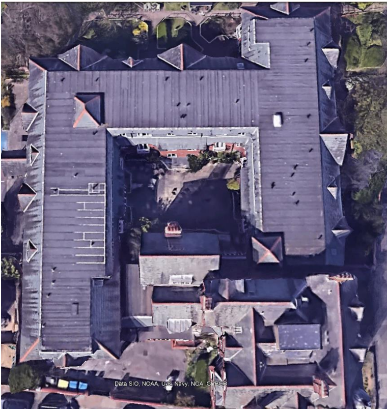
Google Earth view: Showing later extensions on east and north and north west sides later to create a courtyard
