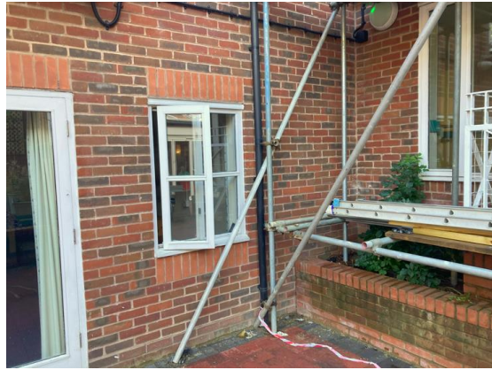
New brickwork on east extension
