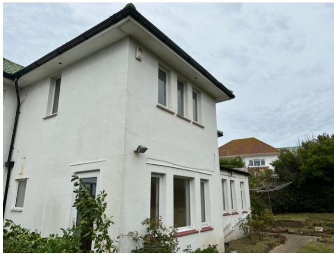
View looking towards part rear elevation of 26 Arundel Drive East
