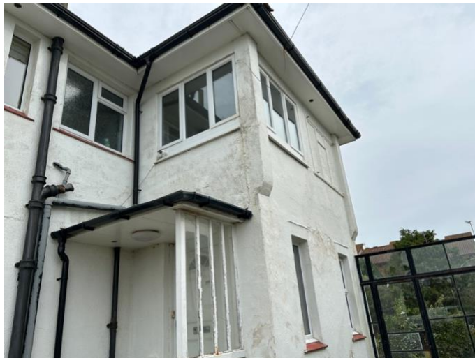
View looking towards south facing side elevation of 26 Arundel Drive East
