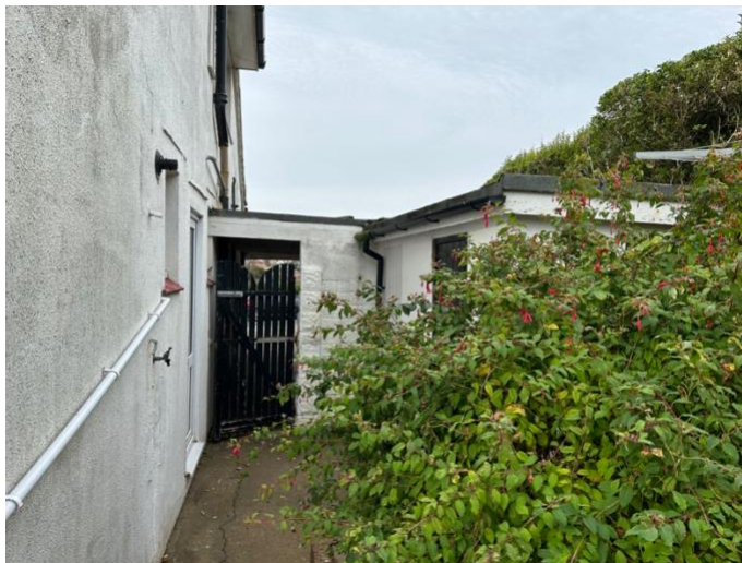
View looking towards north facing side elevation of 26 Arundel Drive East
