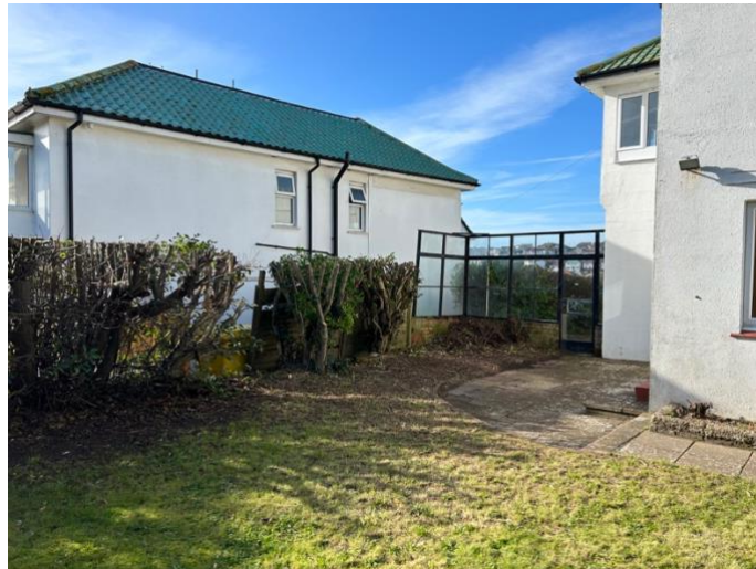
View looking towards the space between number 24 & 26 Arundel Drive East
