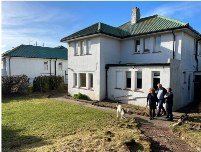
View looking towards rear elevation of 26 Arundel Drive East and side of 24 Arundel Drive East
