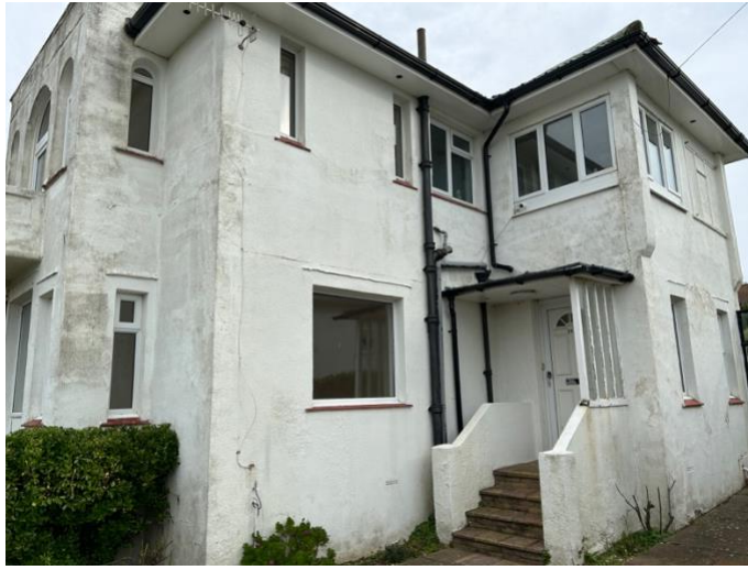
View looking towards south facing side elevation of 26 Arundel Drive East
