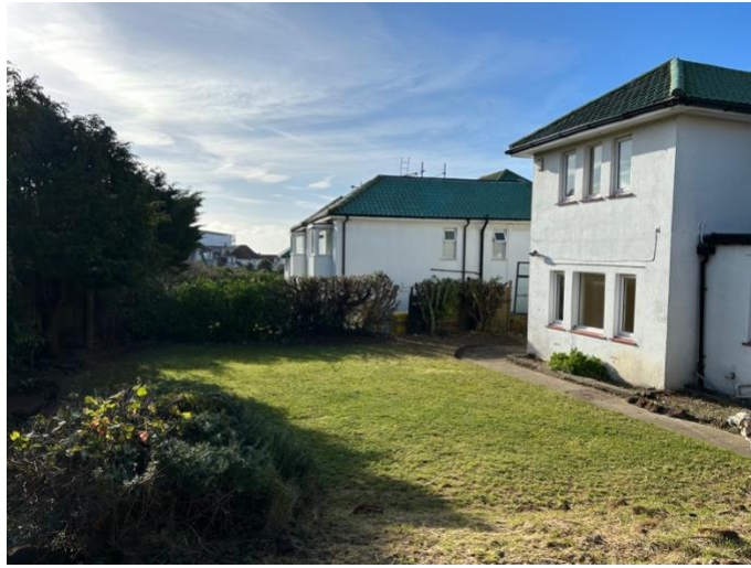
View looking towards part rear elevation of 26 Arundel Drive East and side of 24 Arundel Drive East
