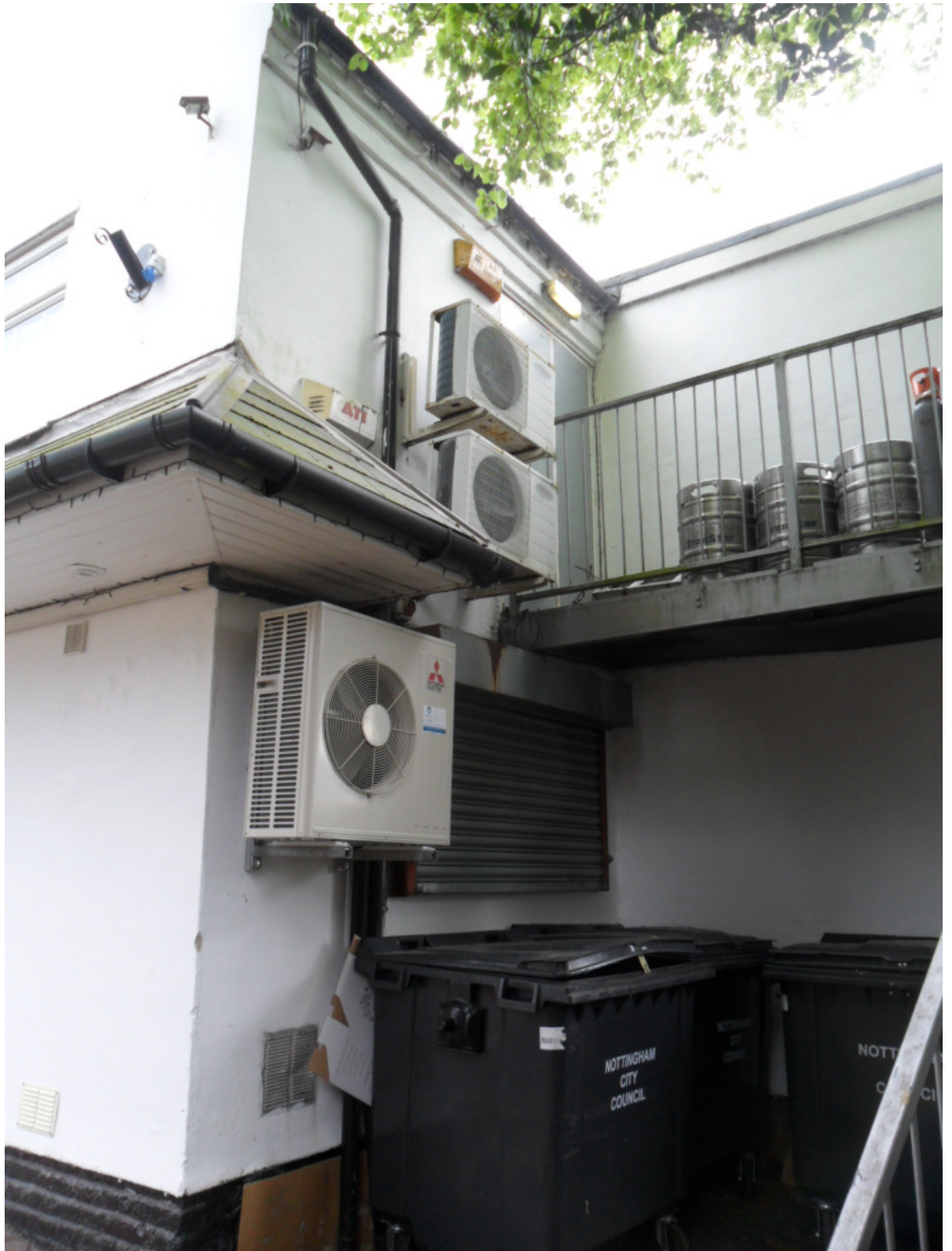
A/C EQUIPMENT AND FIRE ESCAPE since REMOVED
