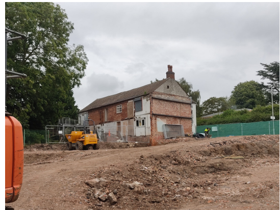
REAR ELEVATION SHOWING ROOF LEVEL DORMER [TANK HOUSING] AND REAR FLAT ROOF EXTENSION [now removed, see photo right]
