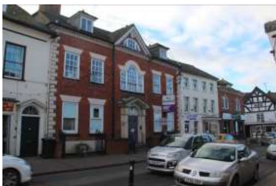
Front/north elevation of 8 Broad Street
