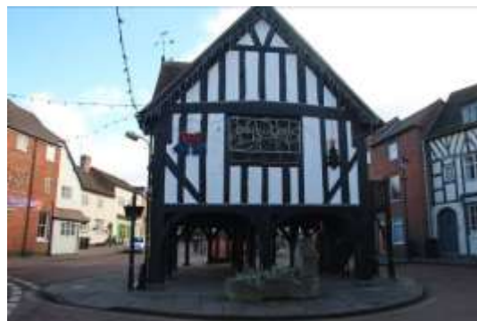
Market Hall northwest elevation – note external staircase to right and stone water trough.
