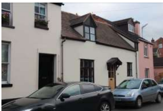
32 Culver Street front elevation
