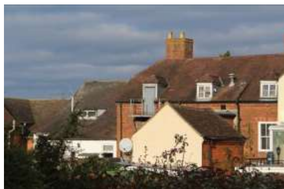
Rear/south elevations of 8 Broad Street from the Site
