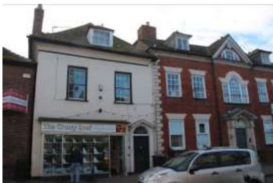
Front/north elevation of 4&6 Broad Street
