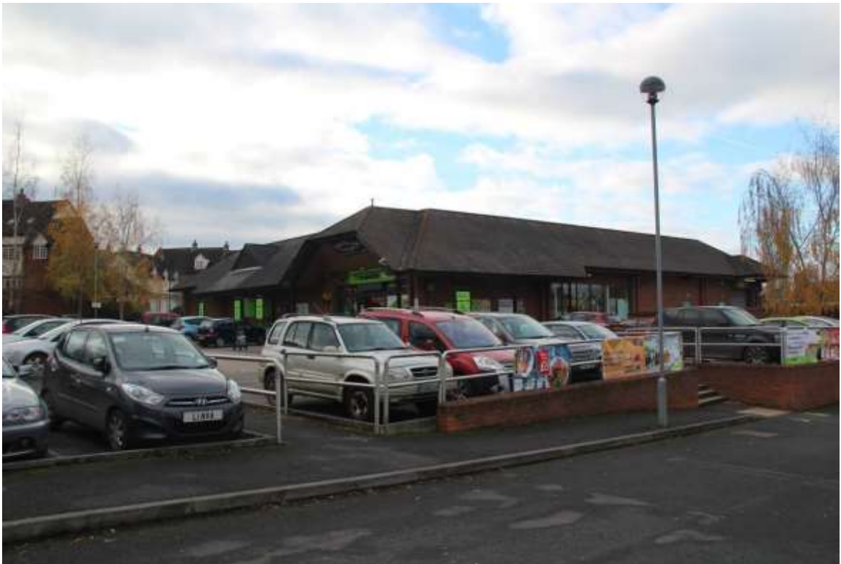
The existing Supermarket – east and north elevations and part of car park from access/servicing road.
