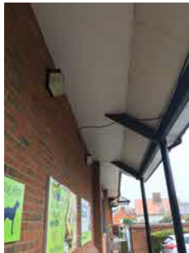
Photograph 14. Overhanging porch and lights
