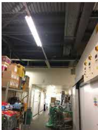
Photograph 19. Warehouse, internal partitions
