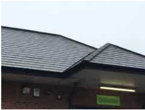
Photograph 13. Clipped gable roof with slate tiles
