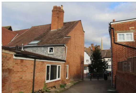
Rear and side of 1 Market Square from the pedestrian footpath.
