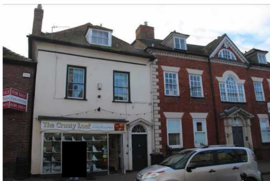
Front/north elevation of 4&6 Broad Street
