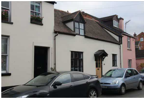
32 Culver Street front elevation
