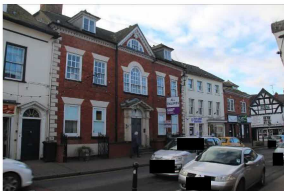
Front/north elevation of 8 Broad Street
