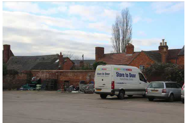
32 Culver Street – part of rear elevation from the Site's Service Yard (No 32 is the property with the lower ridgeline)
