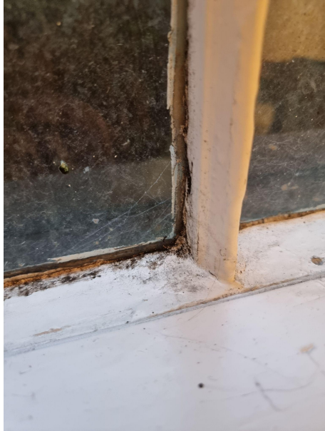
Seals are deteriorating and coming away from the glass. Damage to the internal astragal shows that the wood beneath is soft and rotting.
