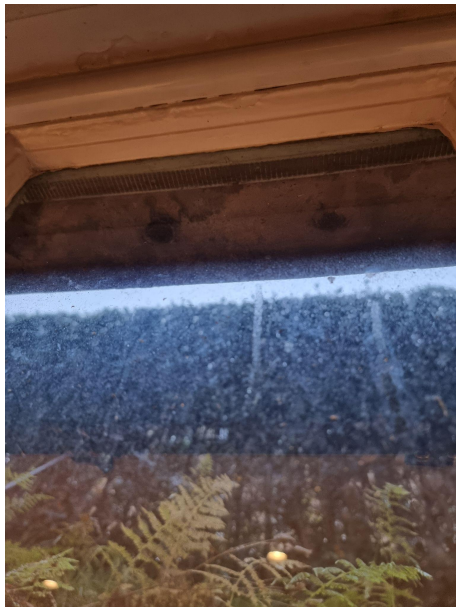
Vents externally to the window are shown in the first photo and the internal dowels are shown in the second photo showing that the windows are not original.
