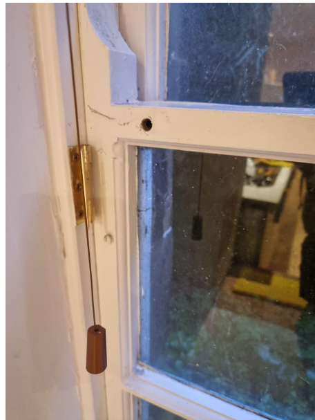
Vents externally to the window are shown in the first photo and the internal dowels are shown in the second photo showing that the windows are not original.
