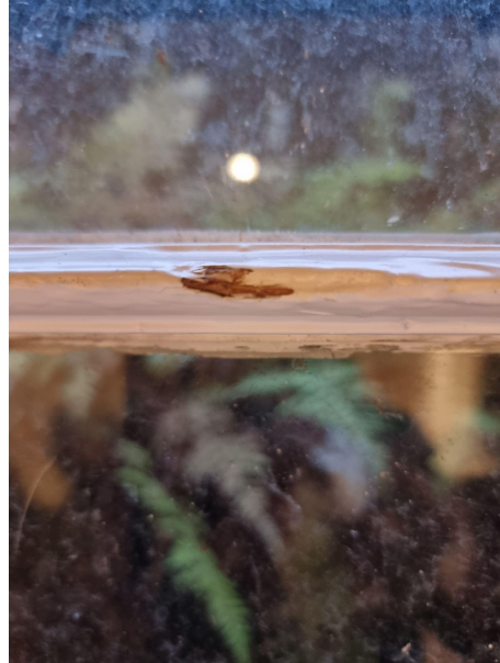
Seals are deteriorating and coming away from the glass. Damage to the internal astragal shows that the wood beneath is soft and rotting.
