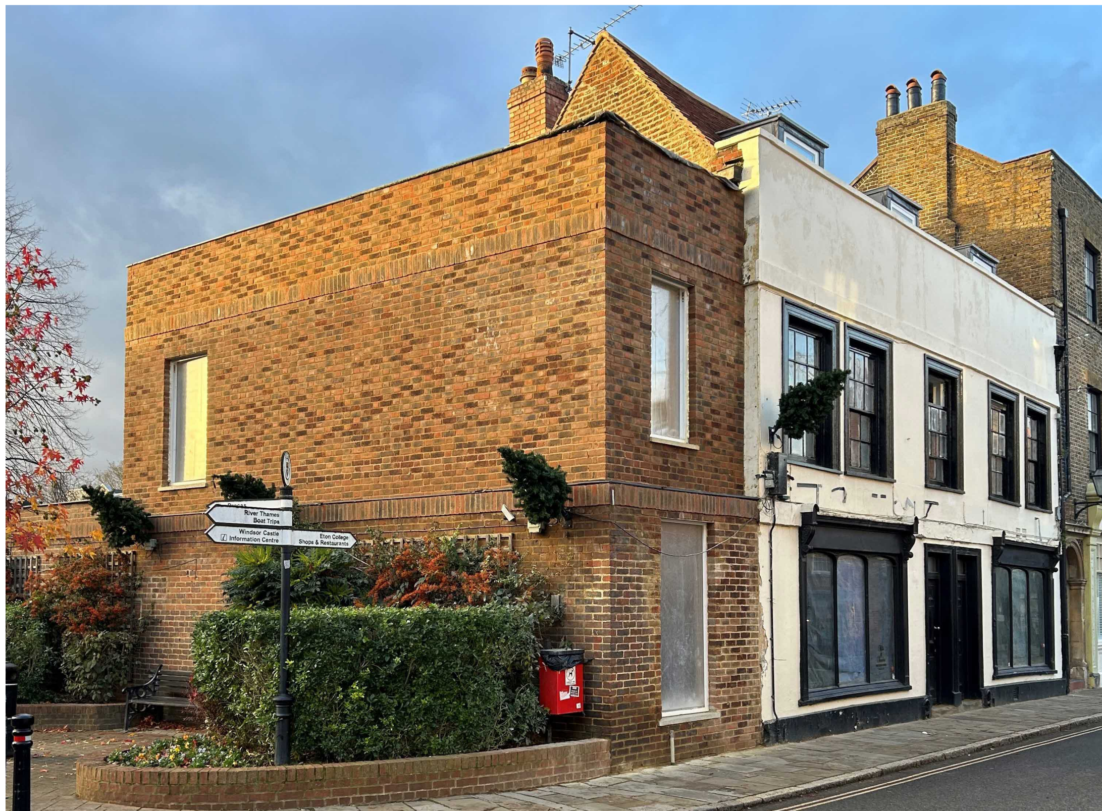
Ongoing building works - November 2023
