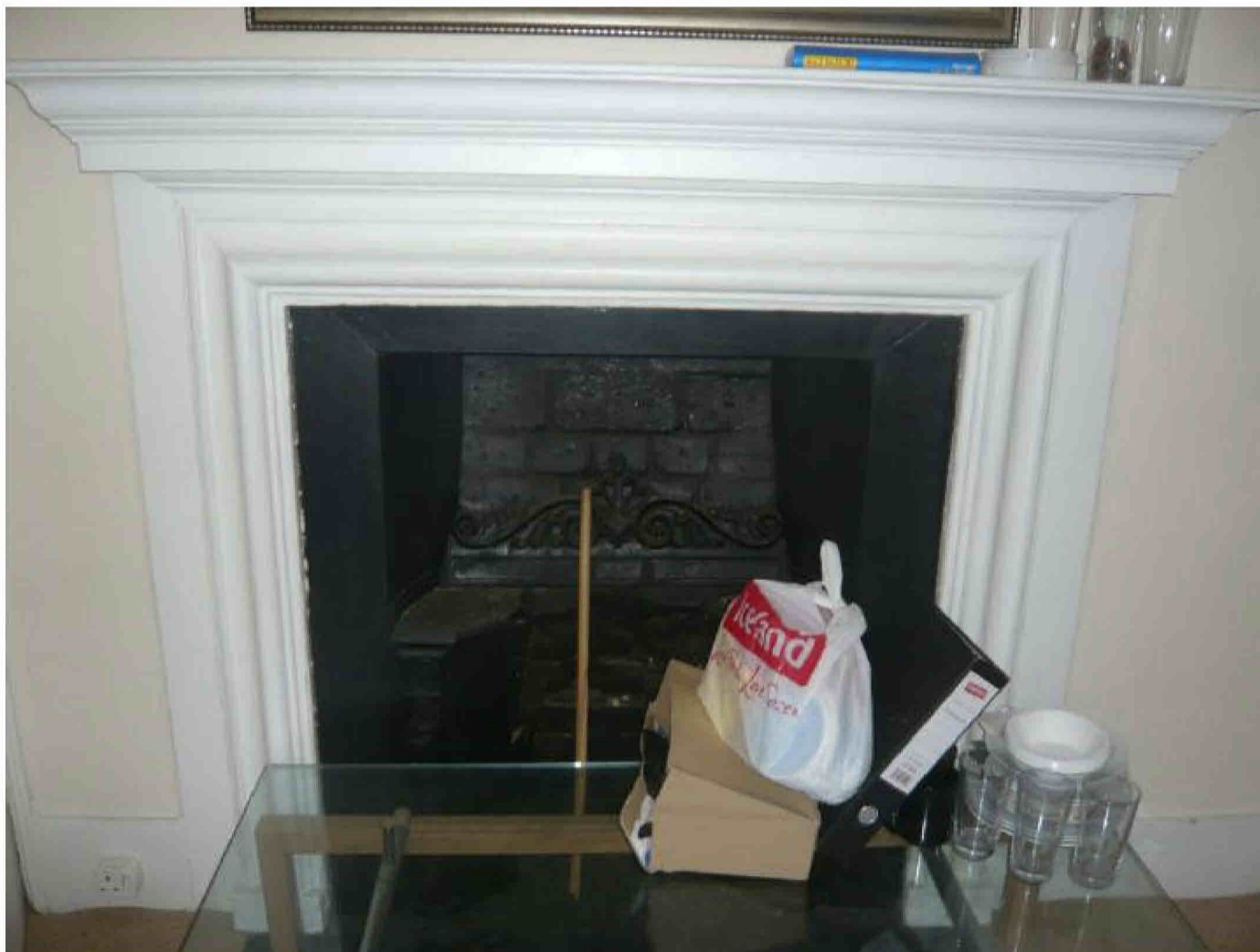
Fig.7 Bolection-moulded fireplace on the first floor
