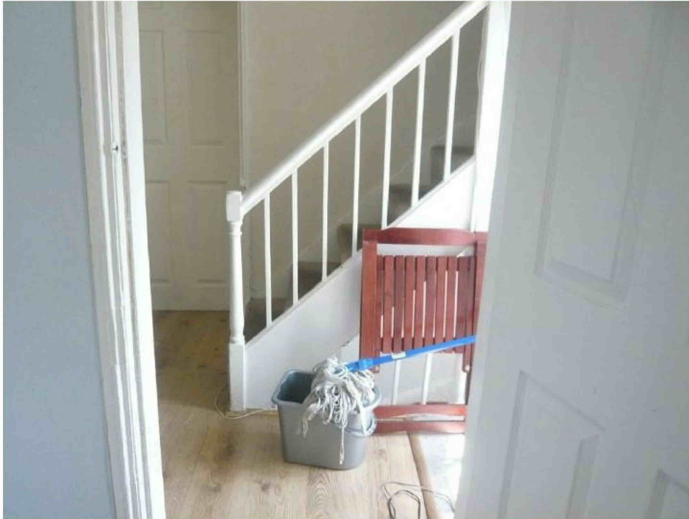
Fig.10 The staircase at the southern end of the first floor
