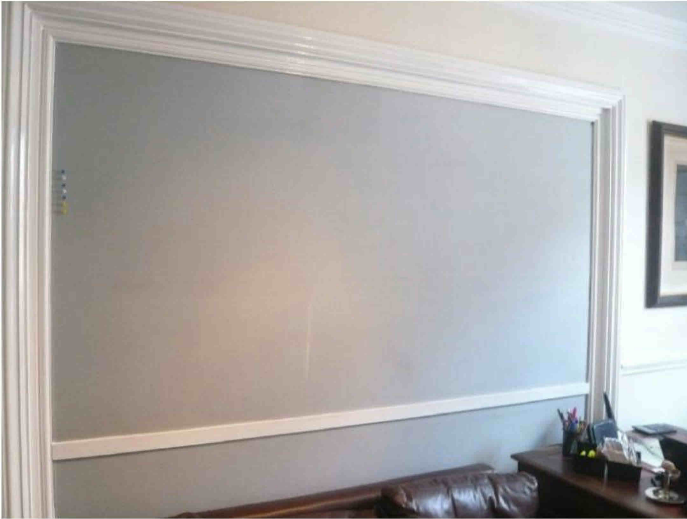
Fig.8 Filled in former wide opening between two first floor rooms
