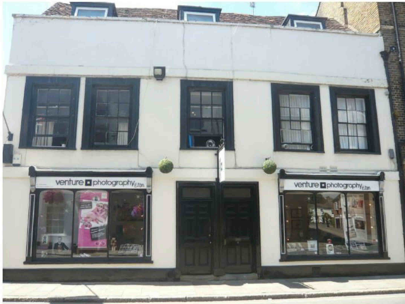
Fig.2 The frontage of 109 High Street
