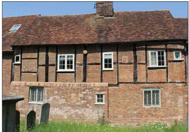
Plate 6. South elevation, looking North
