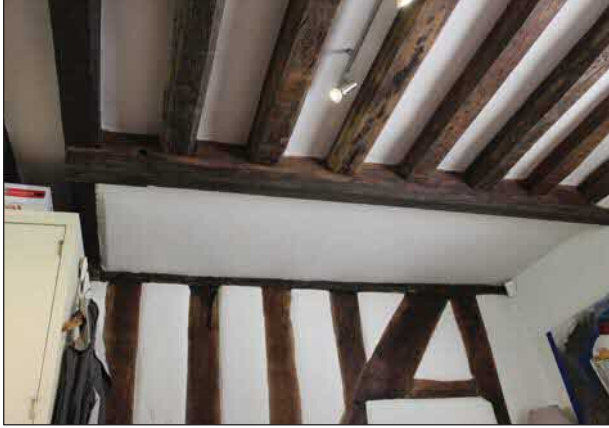
Plate 21. Former stair opening in kitchen, looking East.
