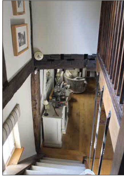
Plate 22. Stair and beam detail, looking West.
