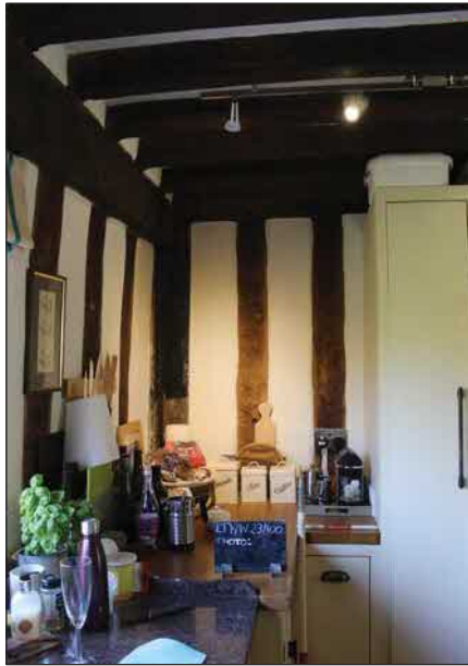
Plate 17. Kitchen, east wall, north end, looking East, Scales: 1x1m, 1x0.3m
