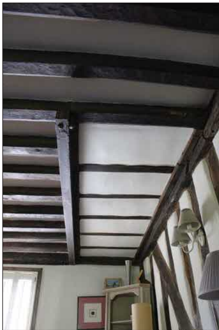
Plate 15. Former stair opening in living room, looking South.
