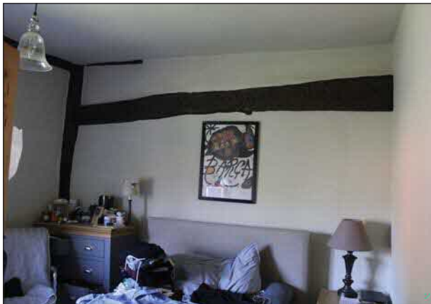
Plate 27. Bedroom 3, east wall, looking East
