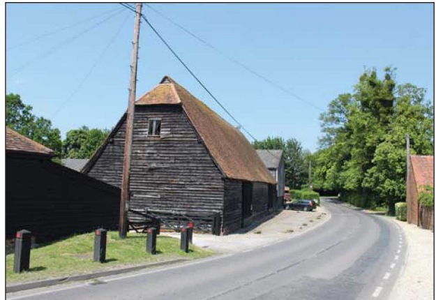
Plate 36. Grade II* barn of Bury Courth, looking Northwest
