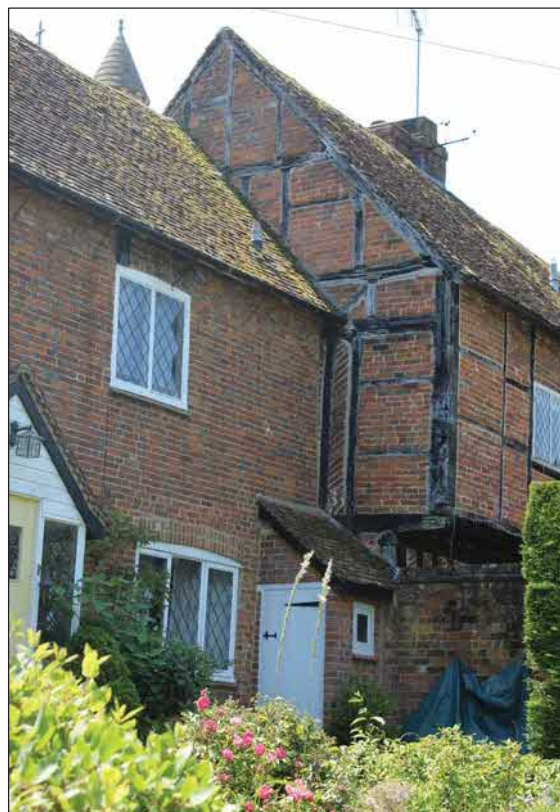
Plate 4. Oblique east elevation, looking south-west
