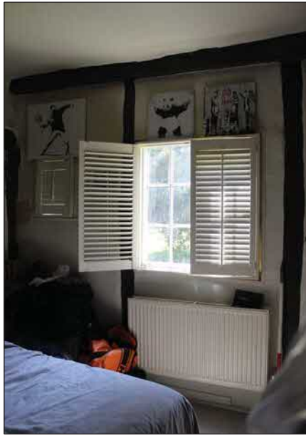
Plate 25. Bedroom 2, joist and beam detail, looking North
