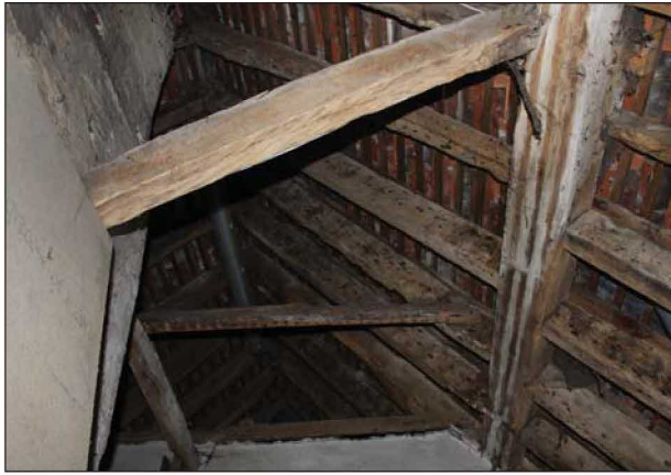
Plate 33. Purlin and rafters, looking West
