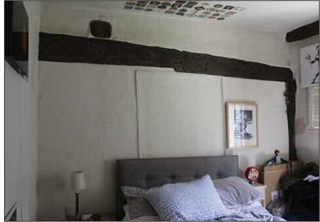
Plate 26. Bedroom 2, east wall, looking East
