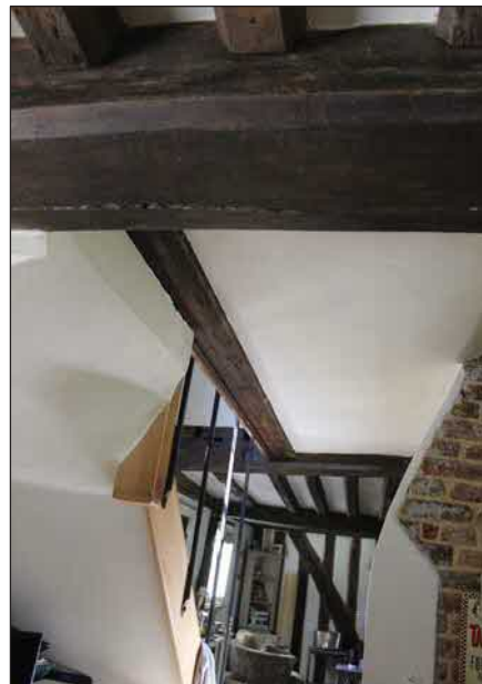
Plate 20. View to living room and stairs, looking West from kitchen.
