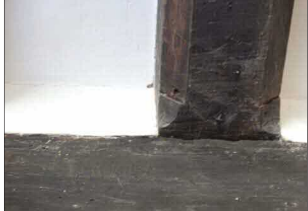
Plate 14. Living room, chamfer and stop joist detail, looking North.
