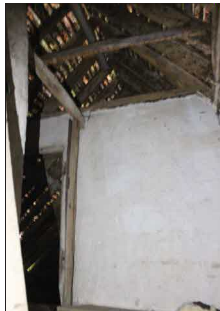
Plate 32. Roof space, west internal wall, looking West
