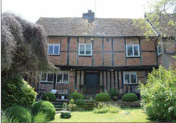
Plate 1. North elevation, looking South, Scale: 1m
