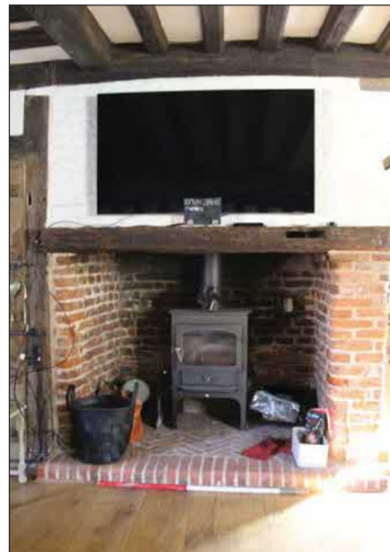
Plate 12. Living room, fireplace detail, looking East, Scales: 1x1m, 1x0.3m
