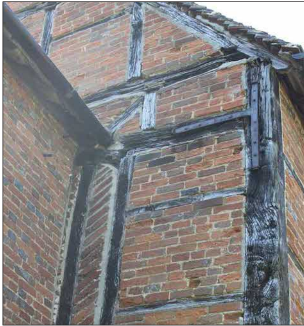
Plate 5. East elevation, looking West
