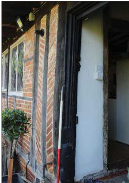
Plate 3. Door jamb detail, looking south-east, Scale: 1m
