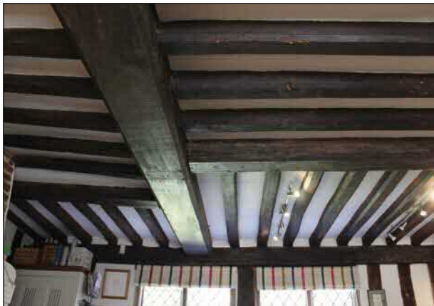
Plate 19. Kitchen ceiling detail, looking North
