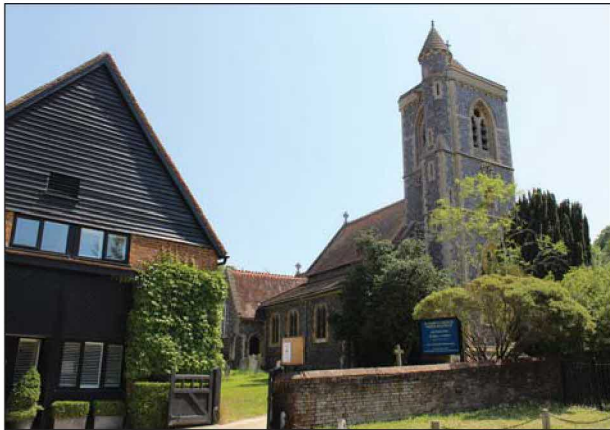
Plate 35. View to church, looking Southeast
