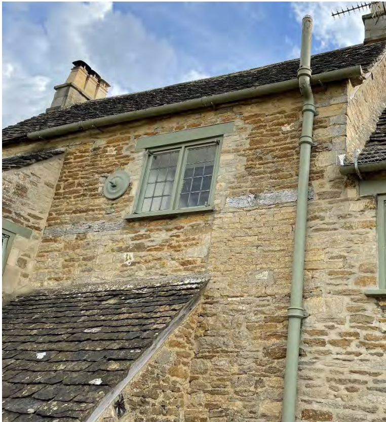
Plate 23: Detail of the rear elevation of the central bays.
