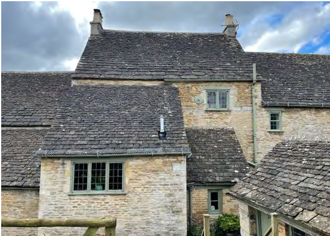
Plate 22: Ampney Brook House, rear extensions to central bays.
