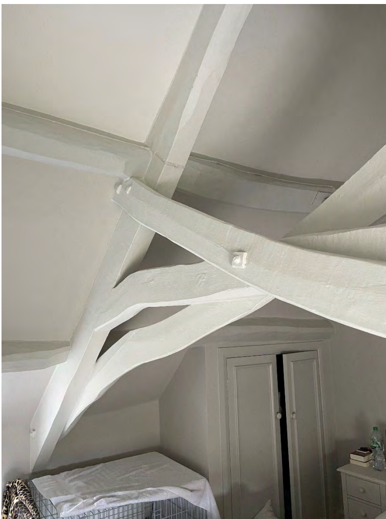
Plate 42: Detail of scissor-type truss in FF18.
