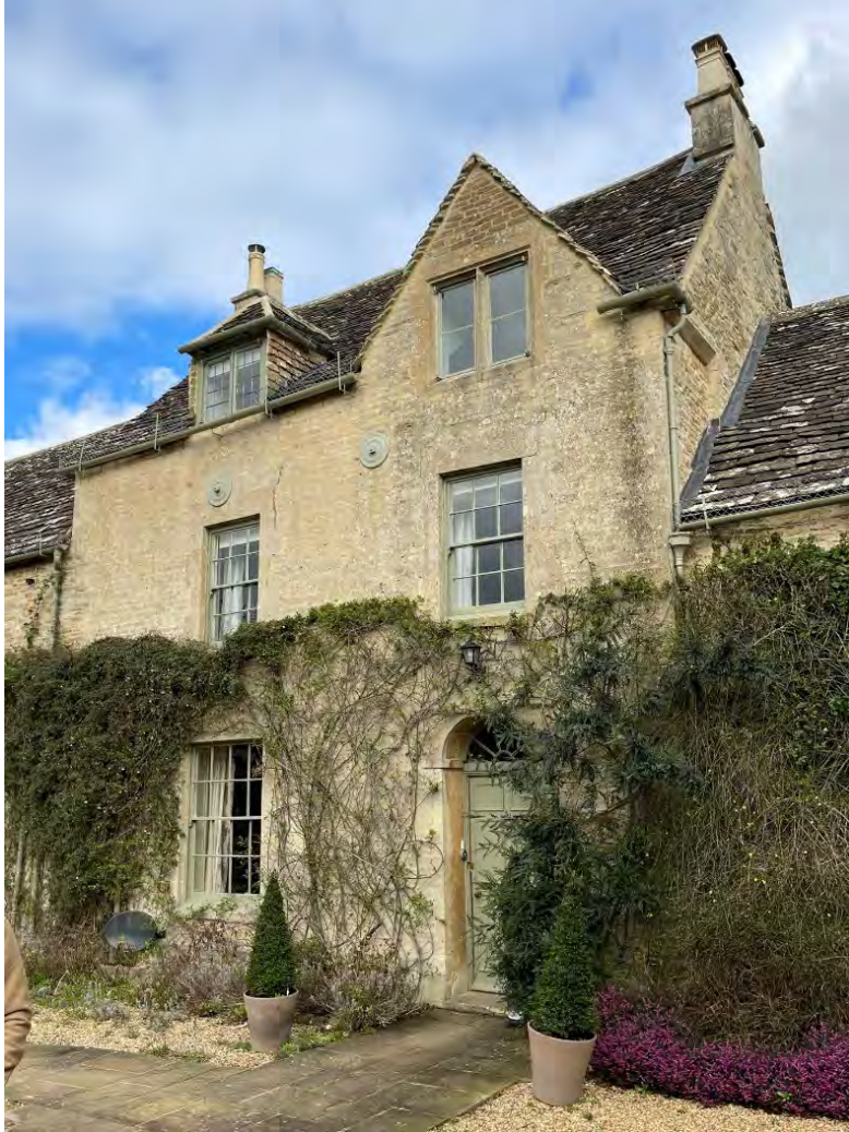
Plate 20: Ampney Brook House, central bays of west range.
