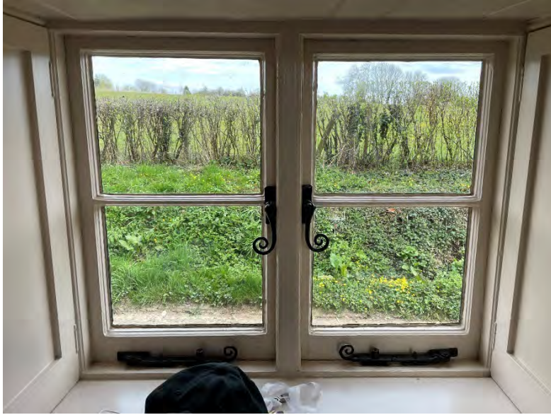
Plate 37: Casement window in east wall of GF10.
