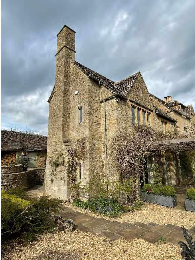
Plate 31: West flank elevation of the main post-war extension.
