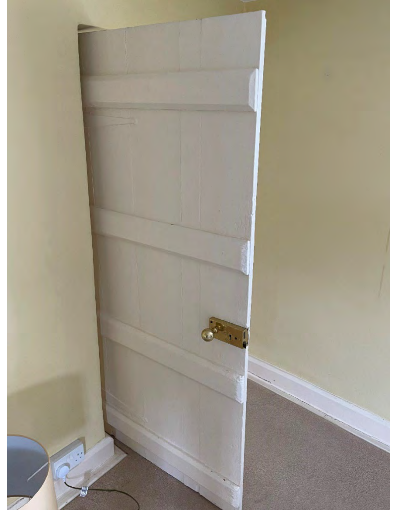
Plate 38: Plank door in FF16.
