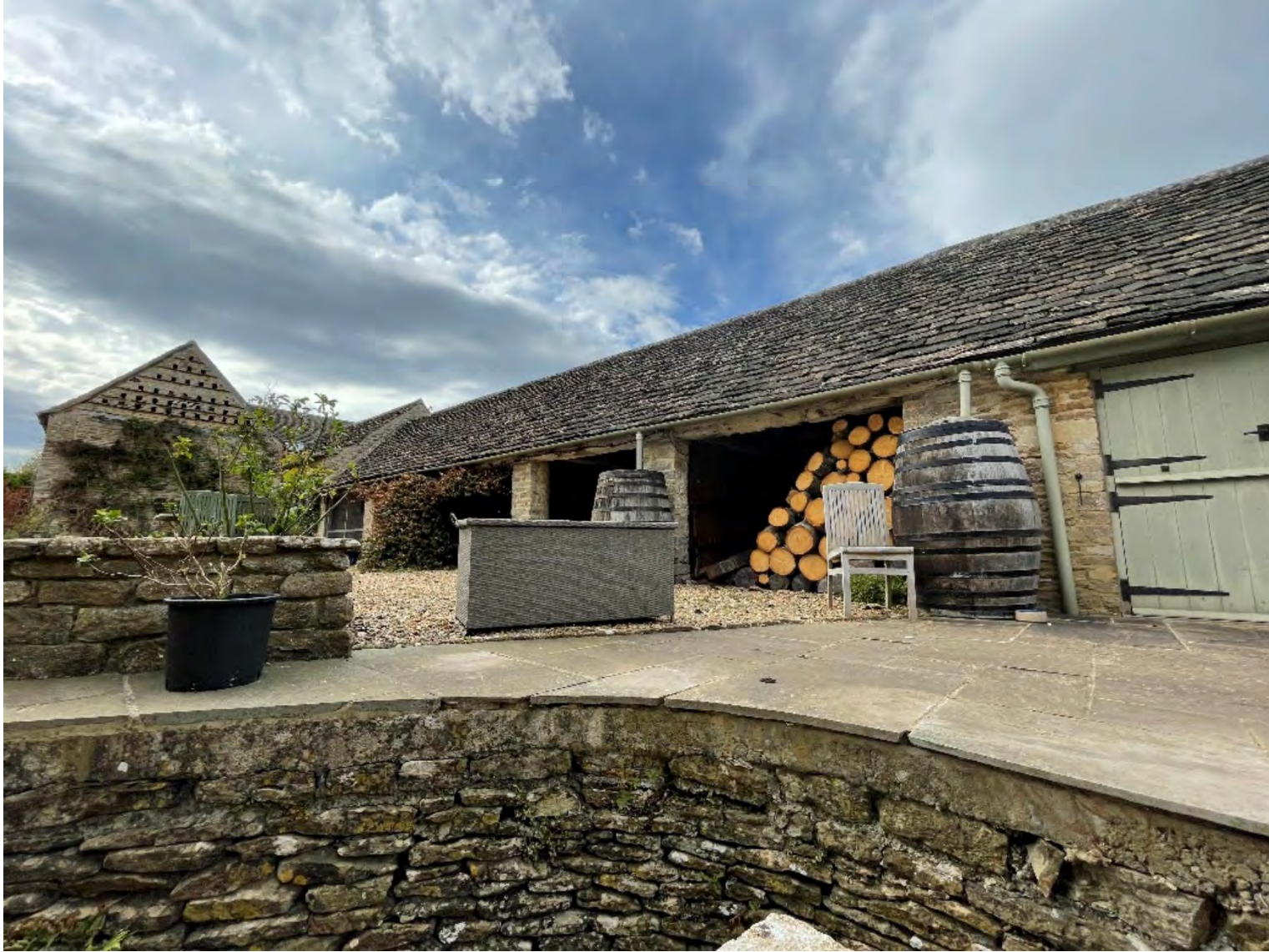
Plate 49: North-west-facing view of the 'cow shed' from the lower level immediately to the rear of Ampney Brook House.
