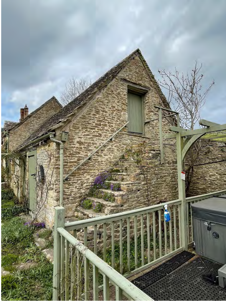
Plate 43: South gable end of the south range.
