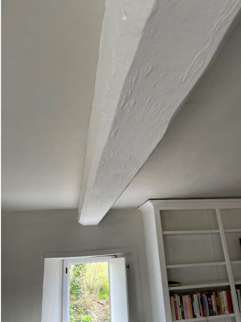
Plate 40: Detail of beam in GF12.
