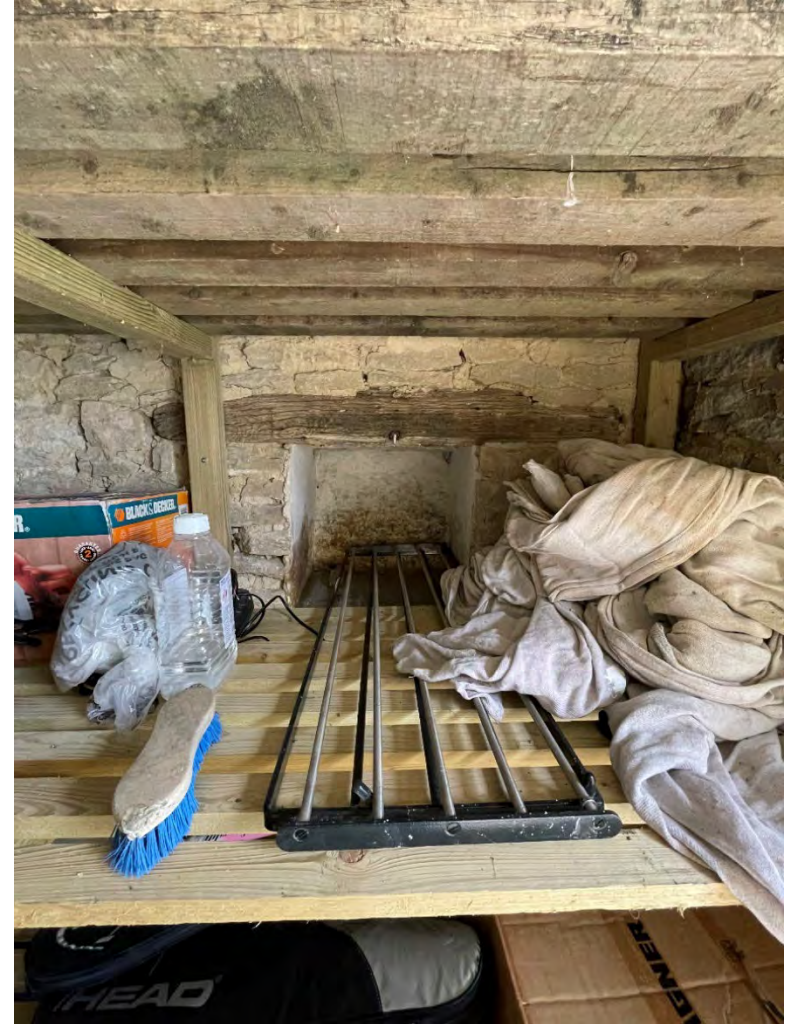
Plate 44: Niche in south wall of GF14.
