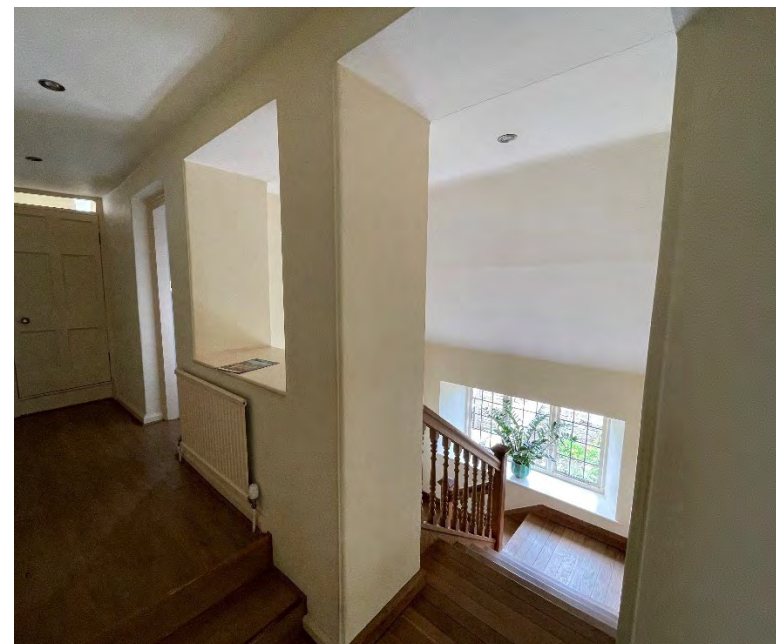
Plate 27: Detail of transition between post-war stairwell and Georgian-style extension.
