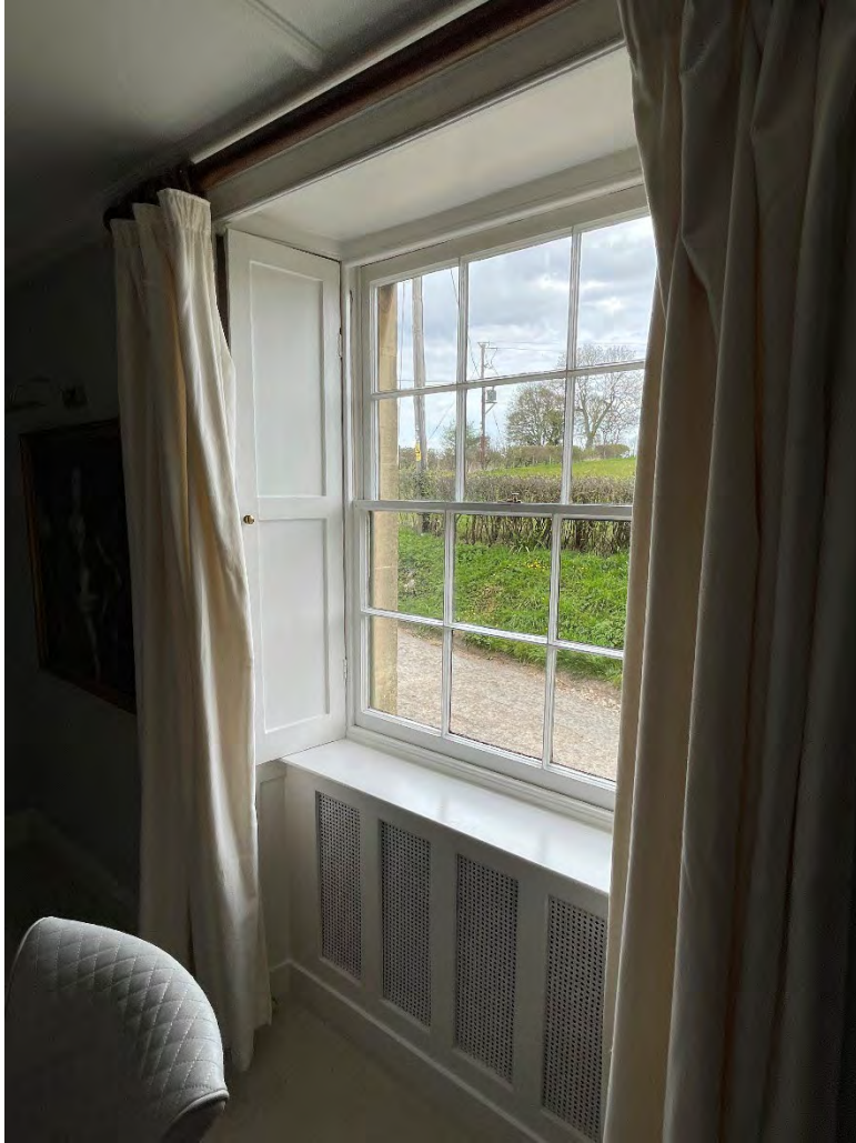
Plate 14: Sash window in east wall of GF6.
