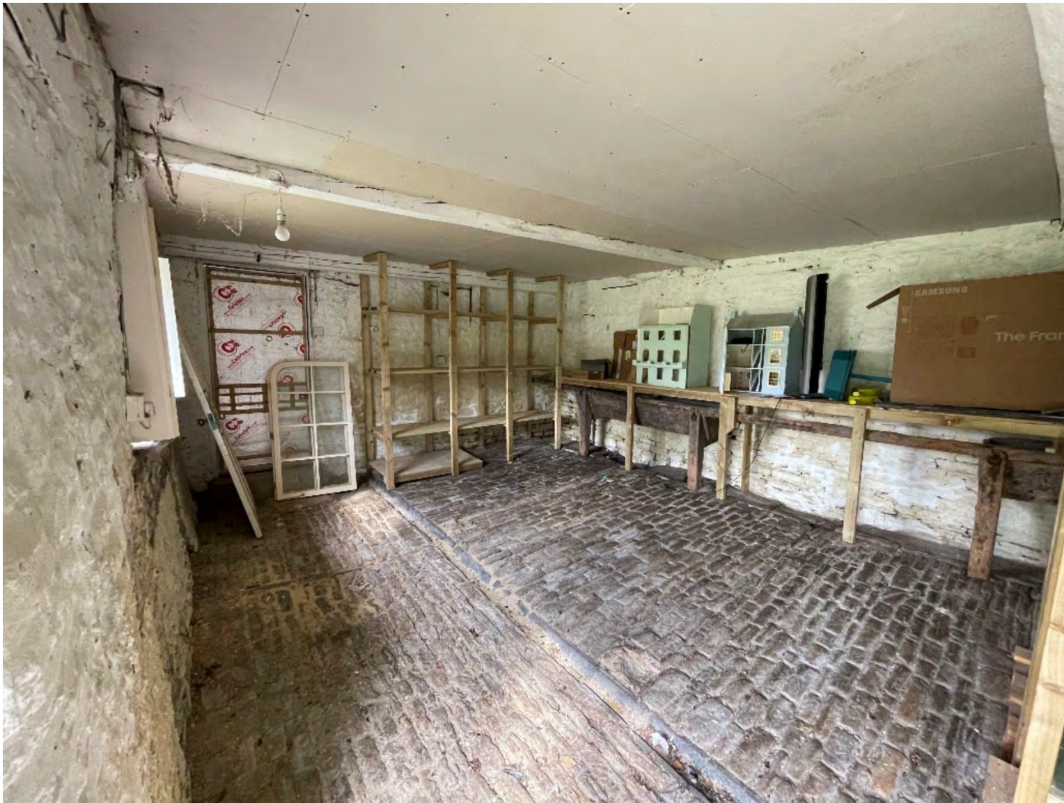
Plate 45: General view of GF13.
