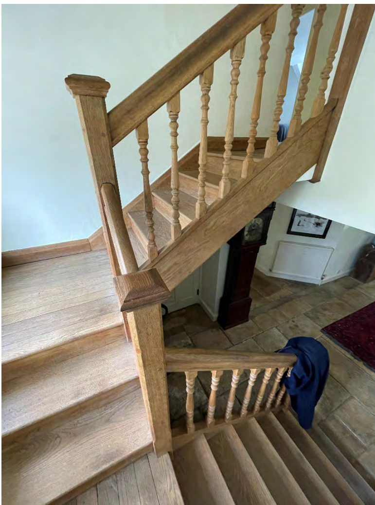
Plate 35: Staircase in rear post-war extension (GF4).
