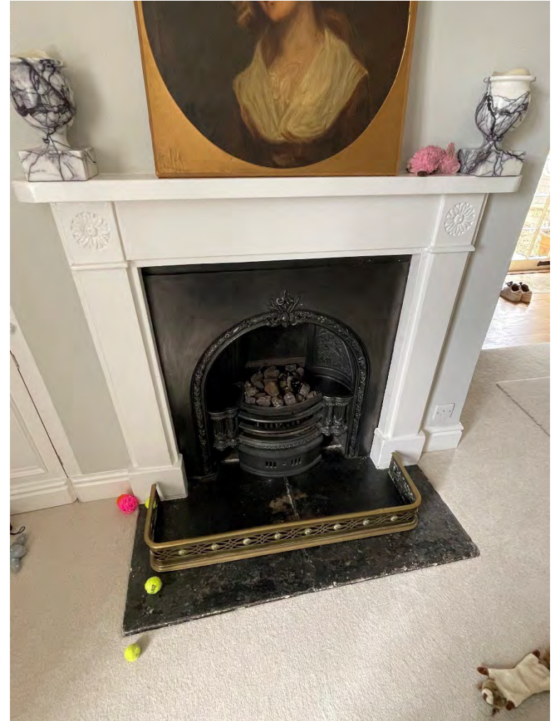
Plate 15: Fireplace in south wall of GF6.
