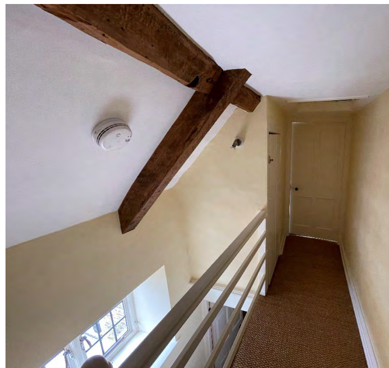
Plate 29: General view of SF1 showing part of exposed roof structure.
