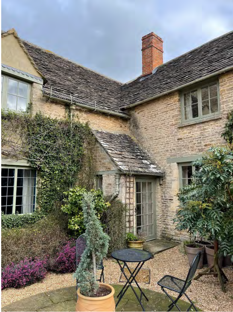
Plate 10: Ampney Brook House, detail of juncture between the west range (left-hand side of frame) and the south range (right-hand side of frame).
