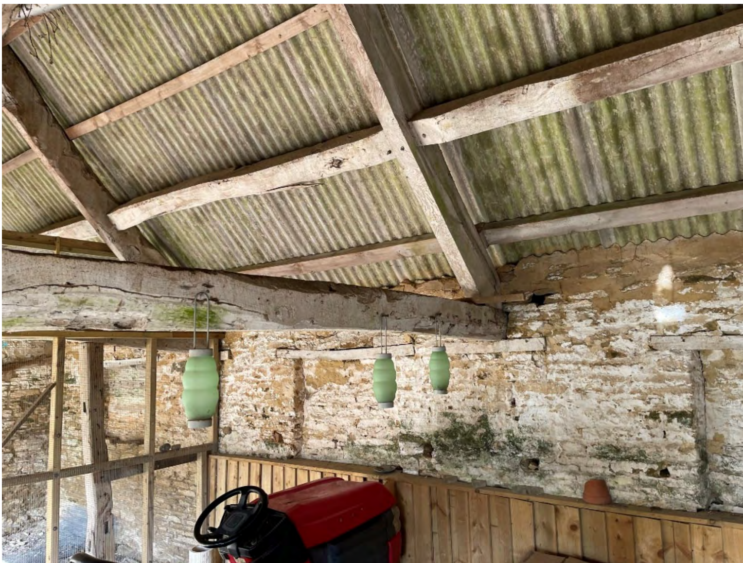
Plate 50: Interior of the 'cow shed', including blocked openings along the north wall.
