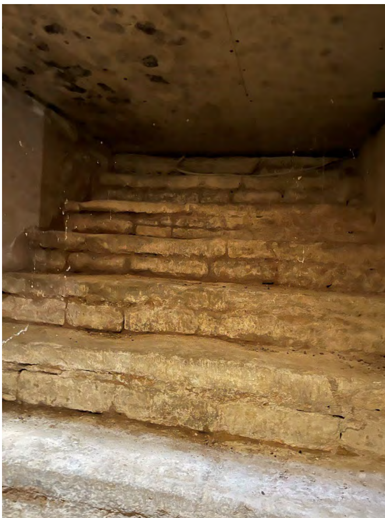
Plate 24: Former stone staircase to cellar (now blocked).
