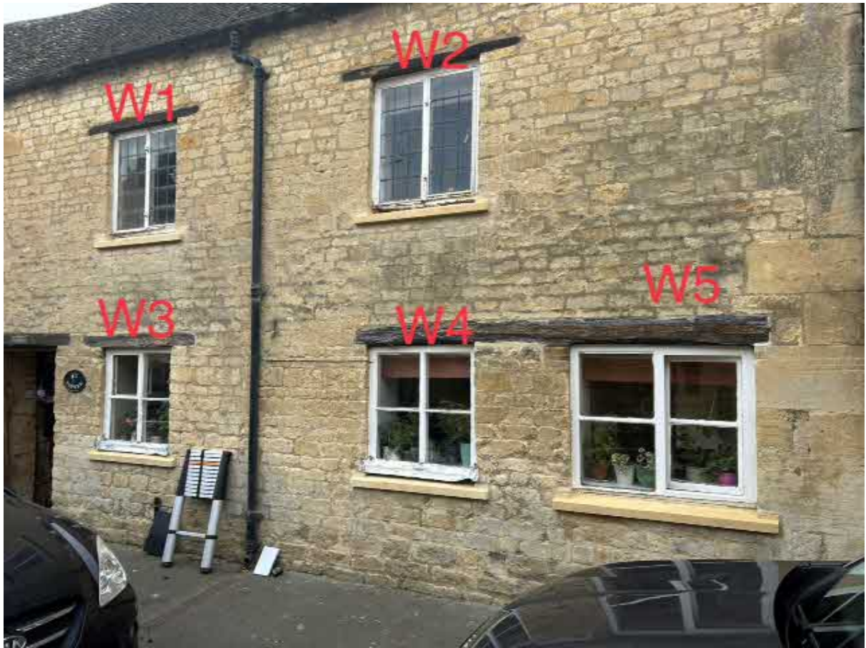
EXISTING FRONT ELEVATION – VIEWED FROM PARK ROAD, SHOWING WINDOW NUMBERS
