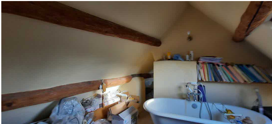
Photograph 6 – bathroom in attic space
