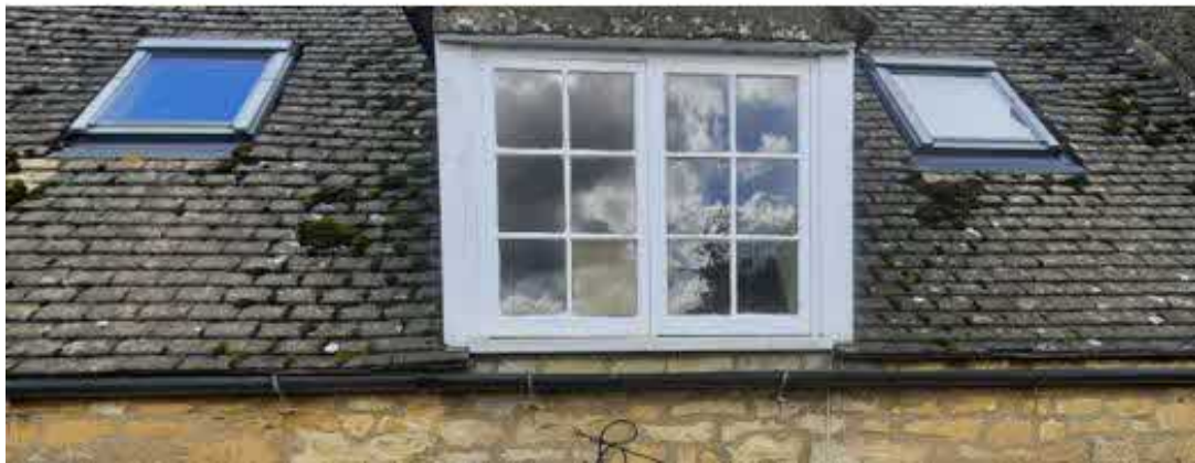
Photograph 7 – dormer window on rear elevation
