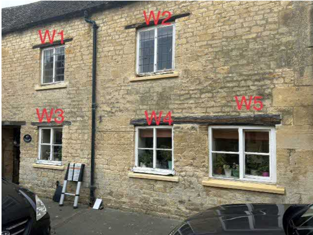
Photograph 8 – Front elevation (after new sills installed), showing window reference numbers
