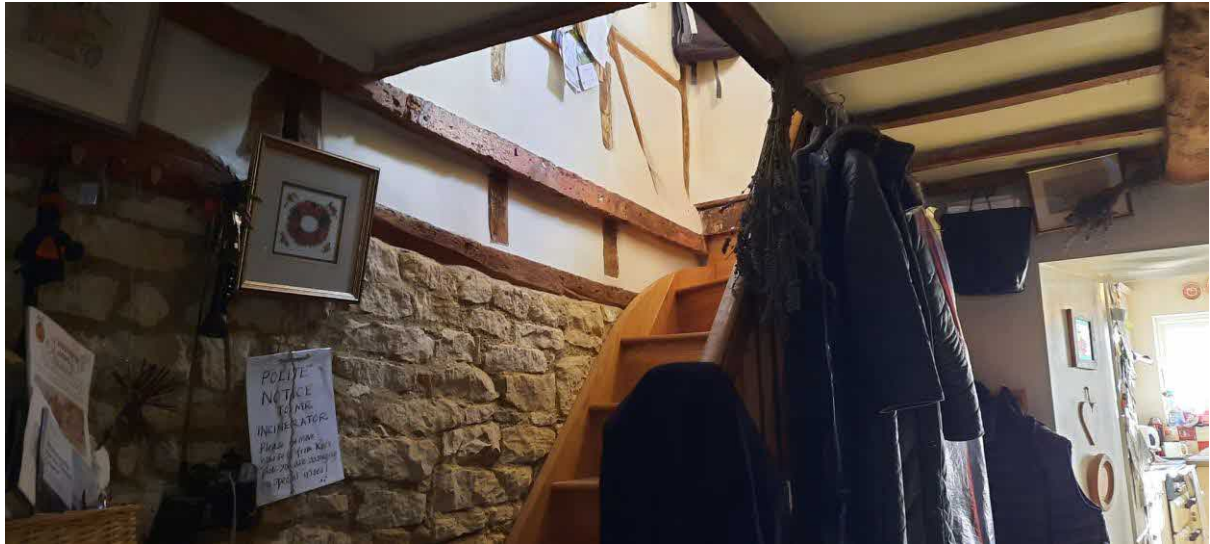
Photograph 7 – hallway showing wattle and daub party wall up the stairs
