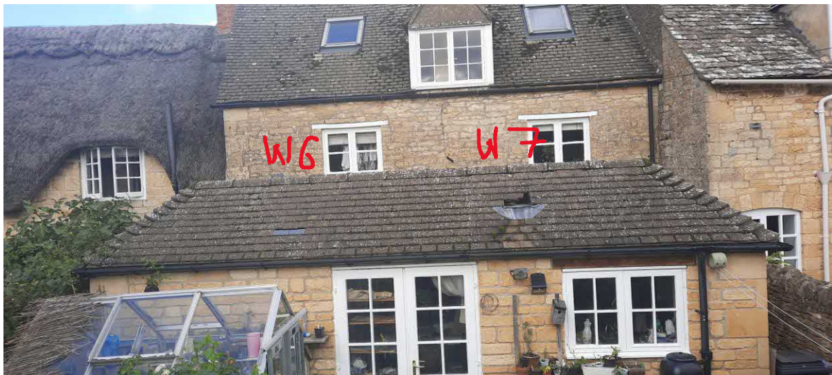
Photograph 9 – Rear elevation, showing window reference numbers
