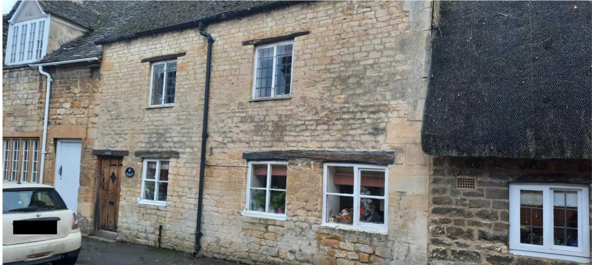
Photograph 1 – Front elevation of Daphne
