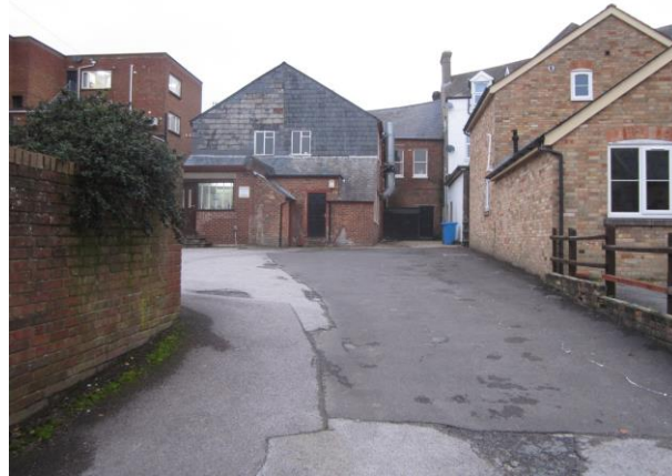
2. The site viewed from Wessex Road.
