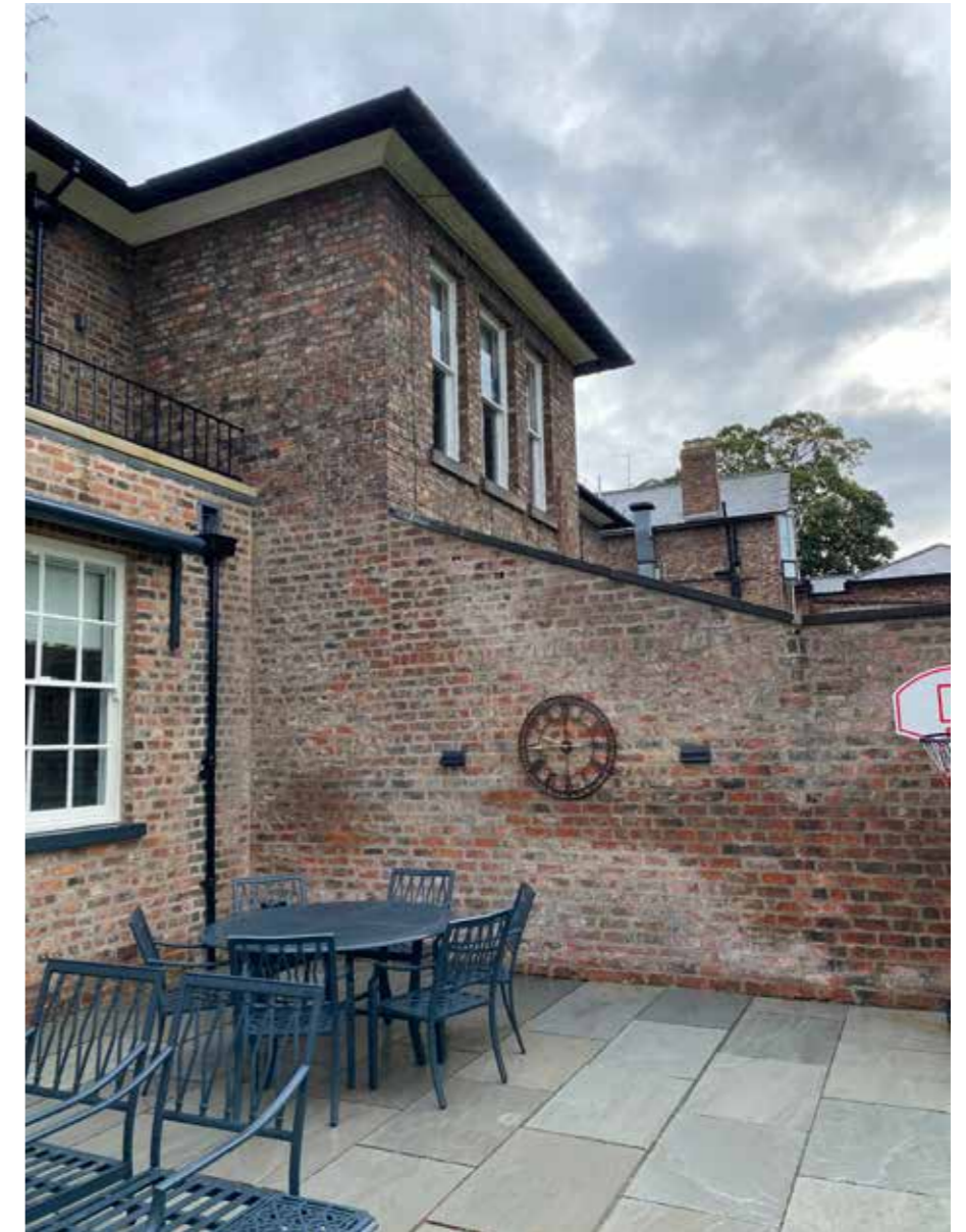
Rear elevation looking towards boundary with 21 Shipton Road
