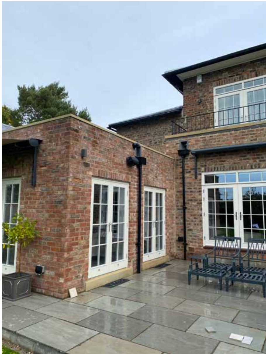
Rear elevation looking towards kitchen/dining area
