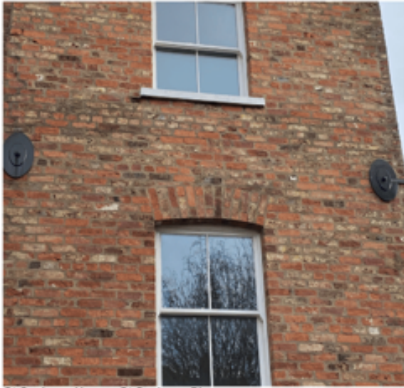
St Saviours House, St Saviours Place
