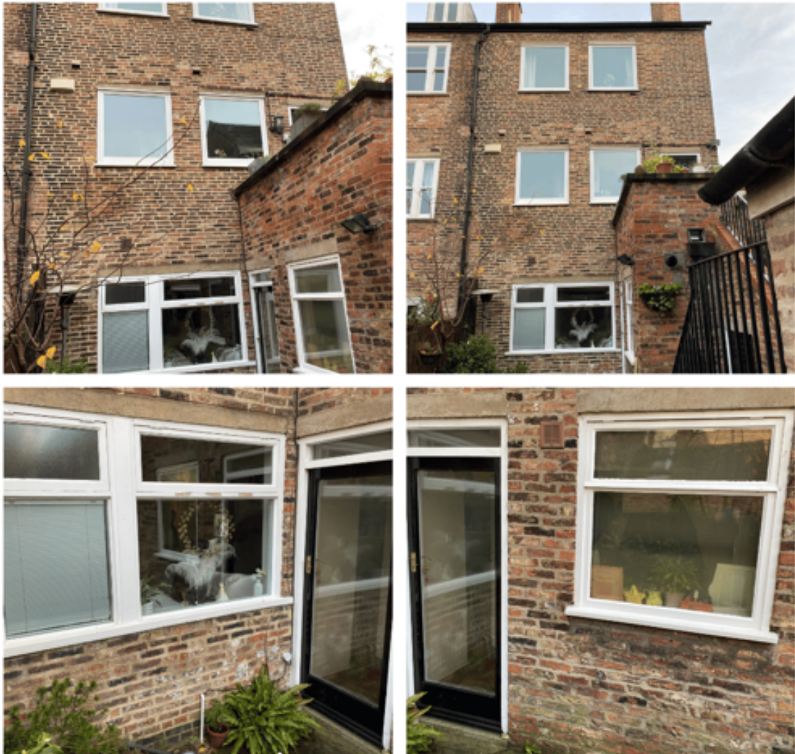
33 St Saviourgate - Existing Rear Elevation, Extension, Doors & Windows
