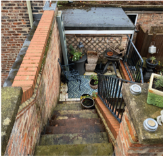
33 St Saviourgate - Existing Roof Terrace & Steps
