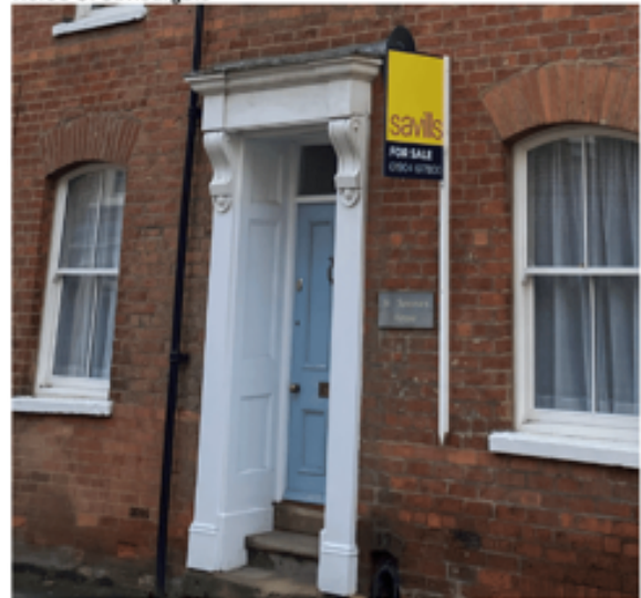
St Saviours House, St Saviours Place
