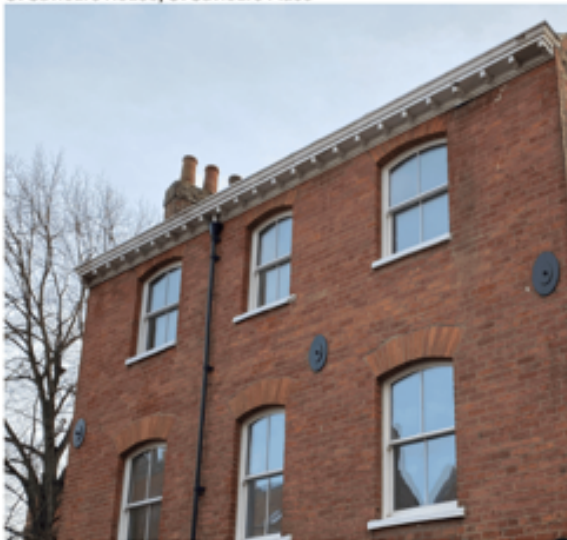
St Saviours House, St Saviours Place
