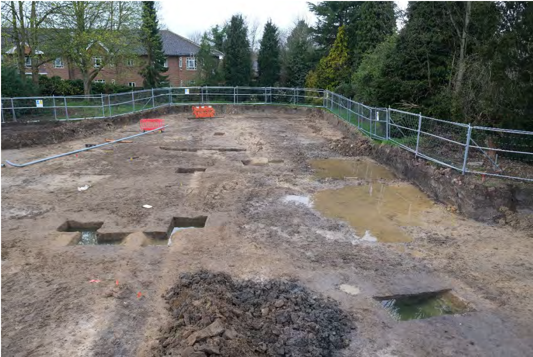
Plate 15 Site overview, facing south-east
