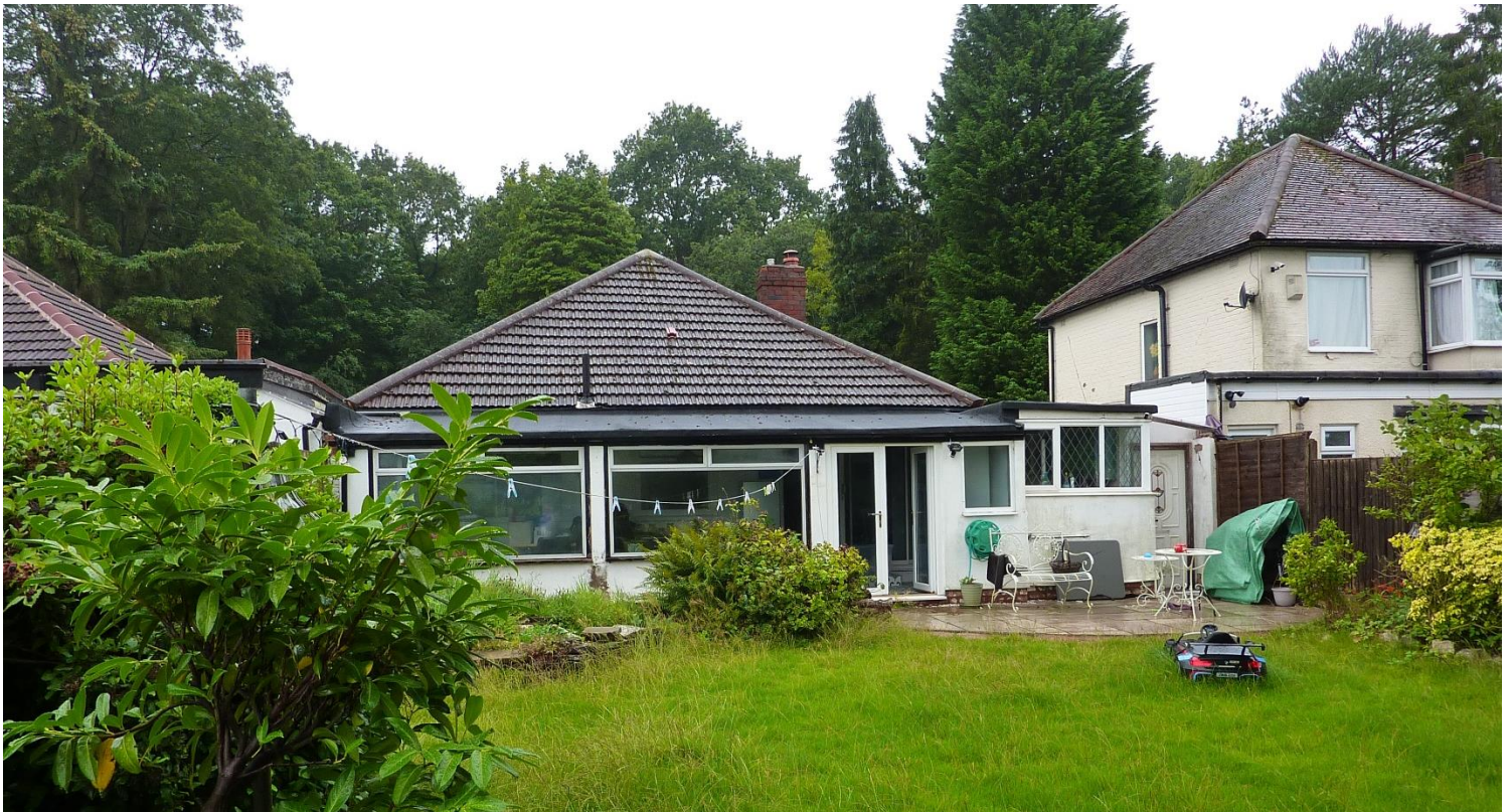
Figure 5. Rear View of the property.
