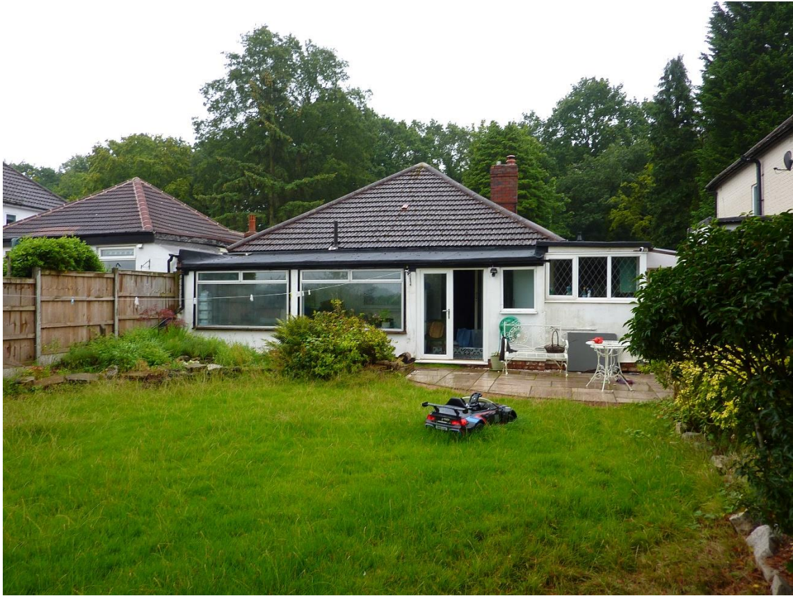
Figure 6: Rear View of the property.
