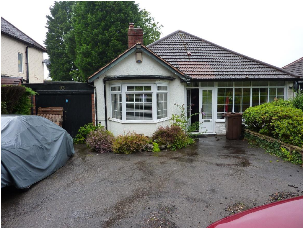
Figure 2: Front elevation of the property, showing the street scene.
