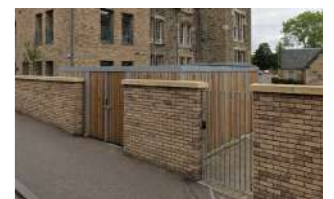
Example of a bin store in Edinburgh with a brick boundary wall and an independent bin store structure behind, with access directly to the street.
