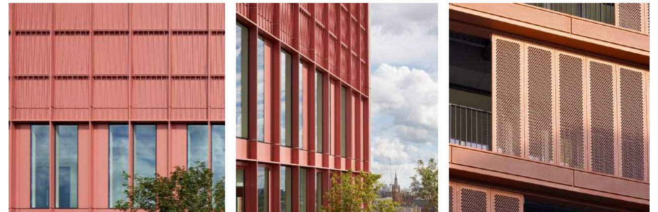
Taylor Maxwell Anvil Metal Cladding System: Allan Murray, New Waverley
