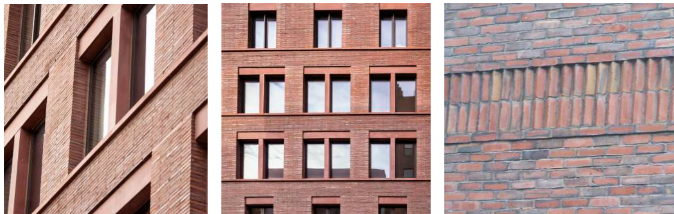
Textured brick with projecting banding: David Chipperfield, New York
