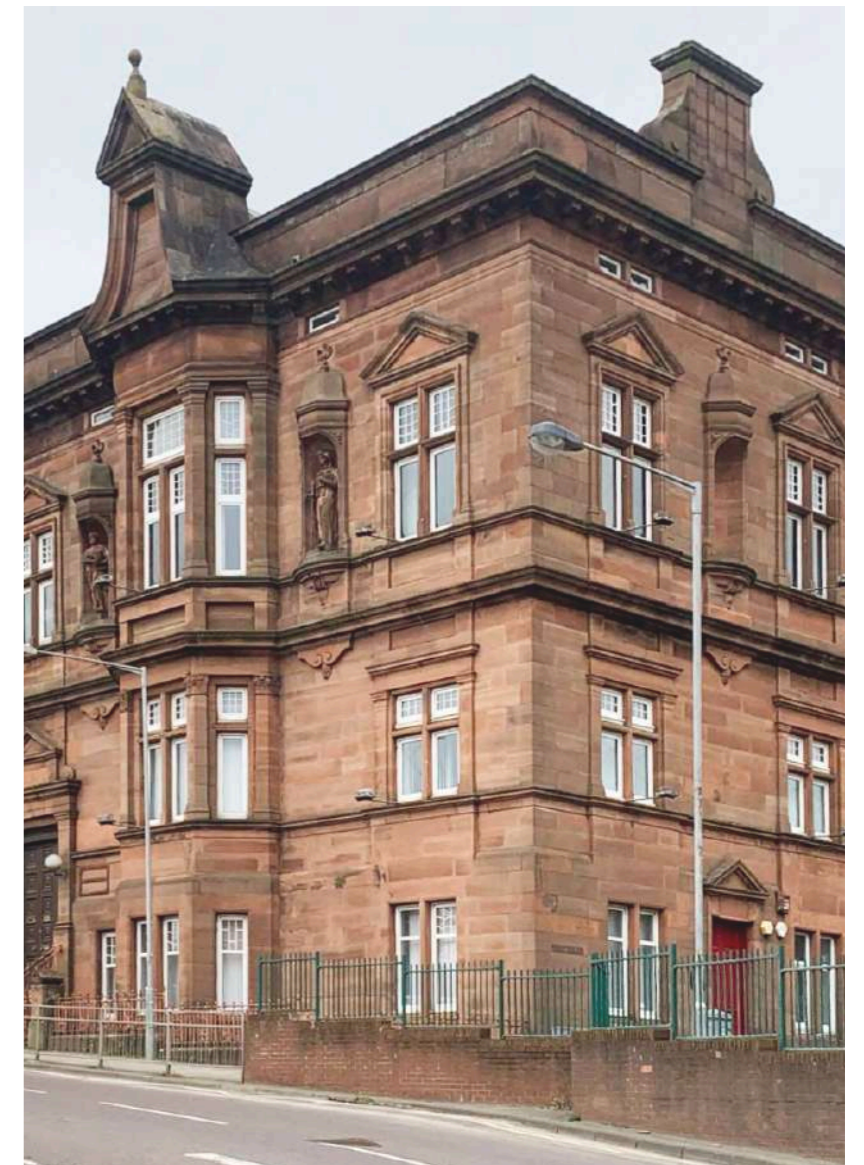
EXISTING MUNICIPAL BUILDING
