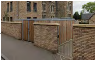
Example of a bin store in Edinburgh with a brick boundary wall and an independent bin store structure behind, with access directly to the street.
