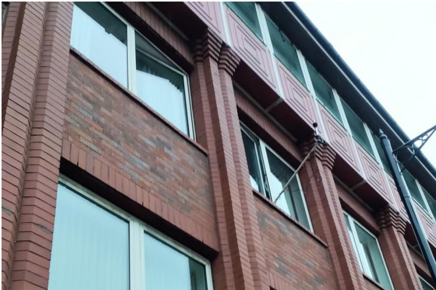
Figure D-1 - Monitoring Position 1, facing North
