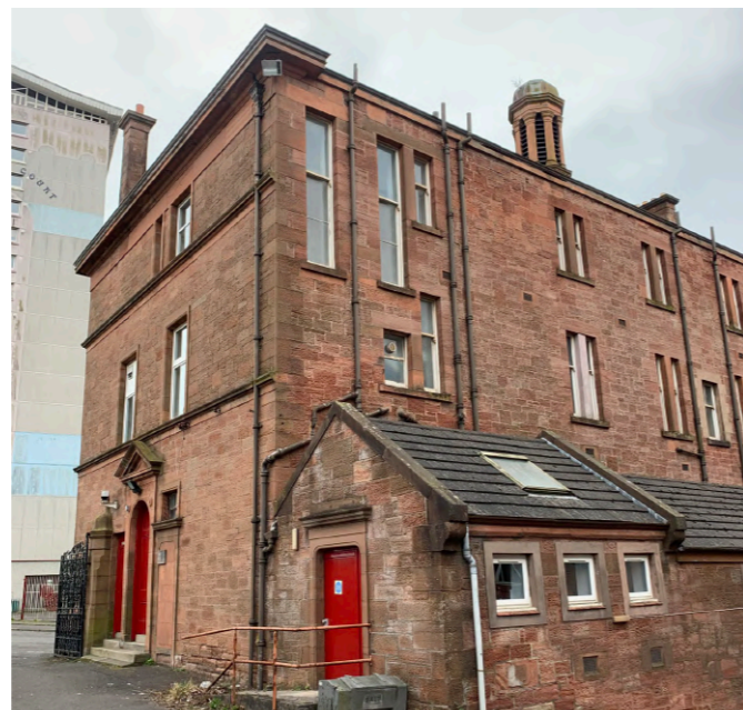
Police wing - external condition
