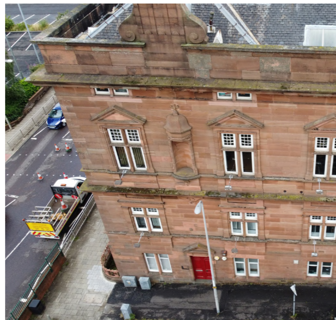
Original victorian wing - external condition
