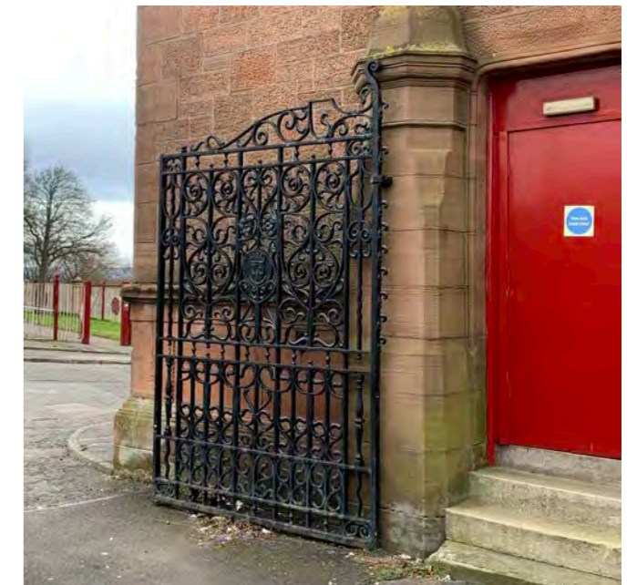
Gateway to courtyard
