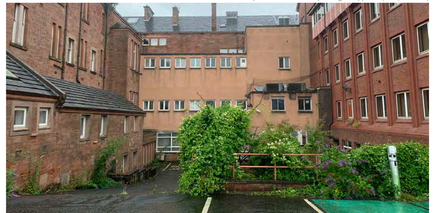
View into East facing courtyard
