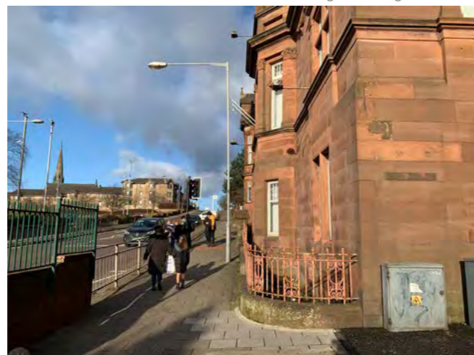
Footpath & external area with hard landscaping along Dunbeth Rd
