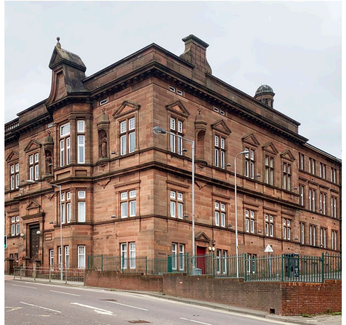
Aerial image of existing Kildonan Street Municipal Building
