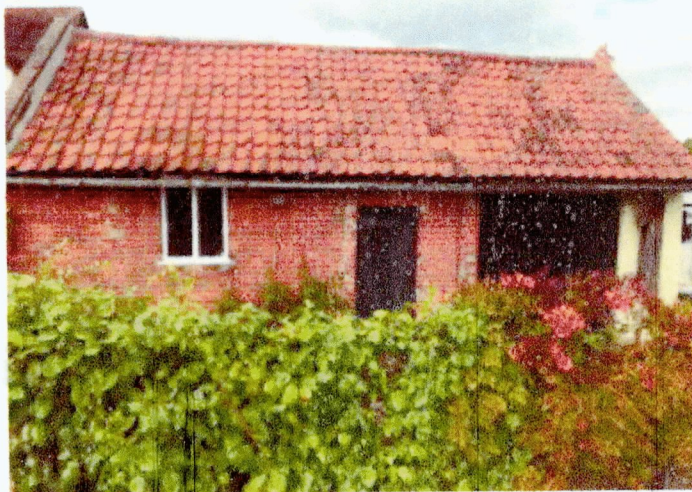
GARAGE SIDE VIEW THE SOLAR PANELS ARE TO GO HERE
