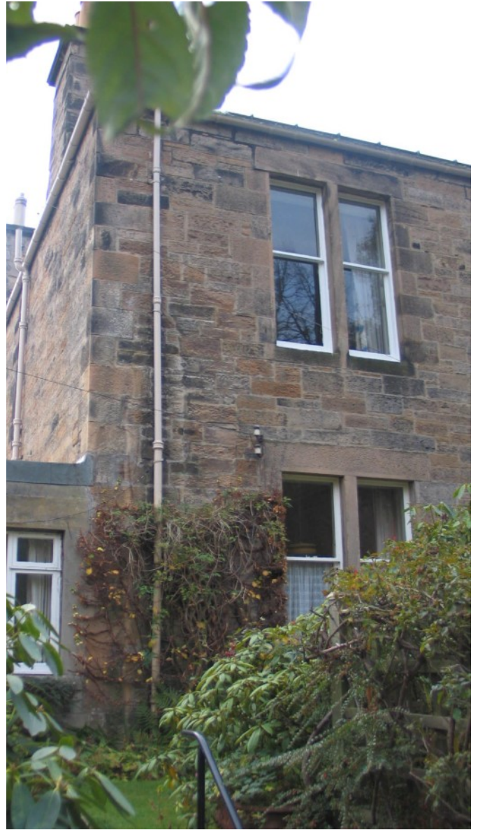
D EXISTING VIEW OF REAR ELEVATION
