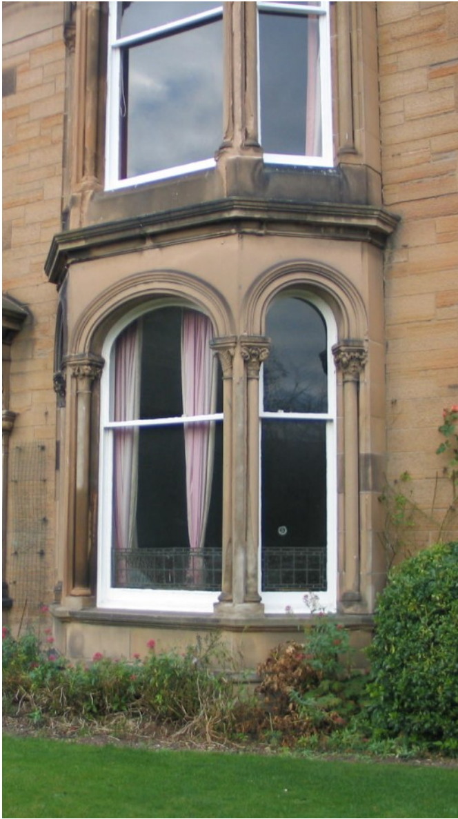
C EXISTING VIEW OF VILLA SHOWING THE LIVING ROOM WINDOW
