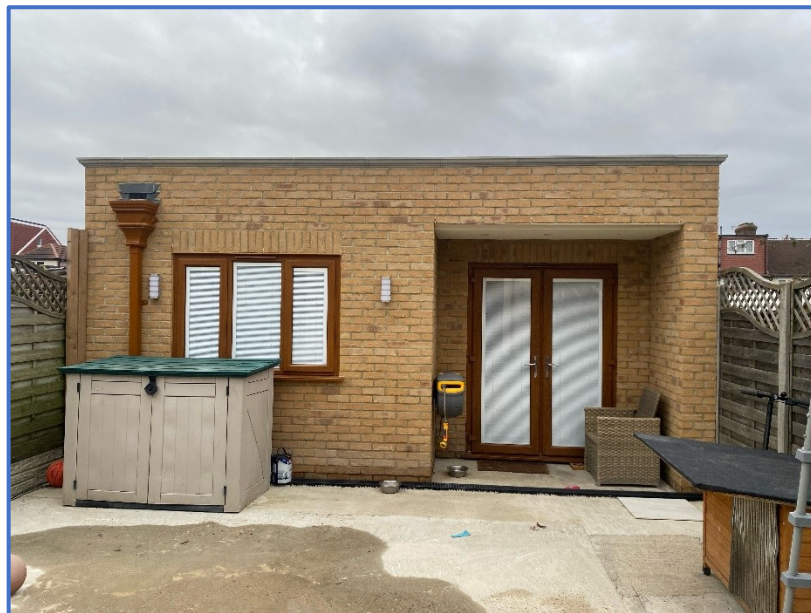
Figure 2 – View of the existing building – front elevation
