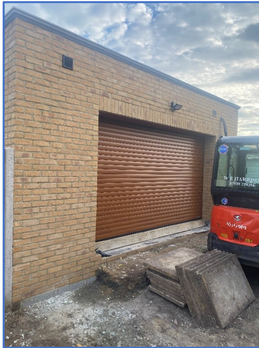
Figure 3 – View of the existing building – rear elevation
