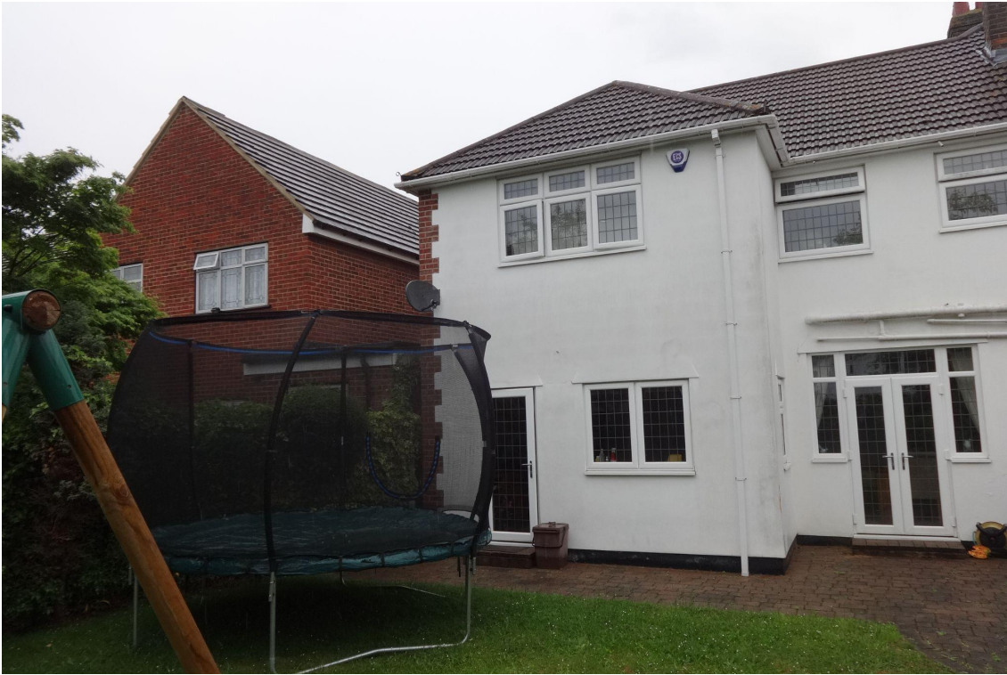
Fig. 1 Existing rear elevation with number 69 Gloucester Avenue (left).
