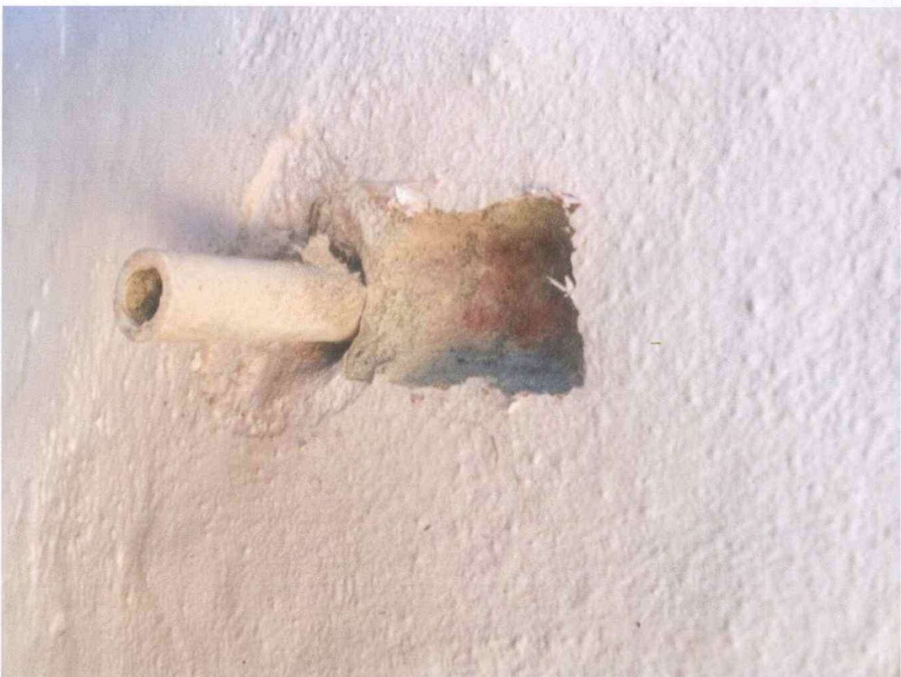
PHOTO 5 BRICK CONSTRUCTION EXTERNAL KITCHEN WALL
