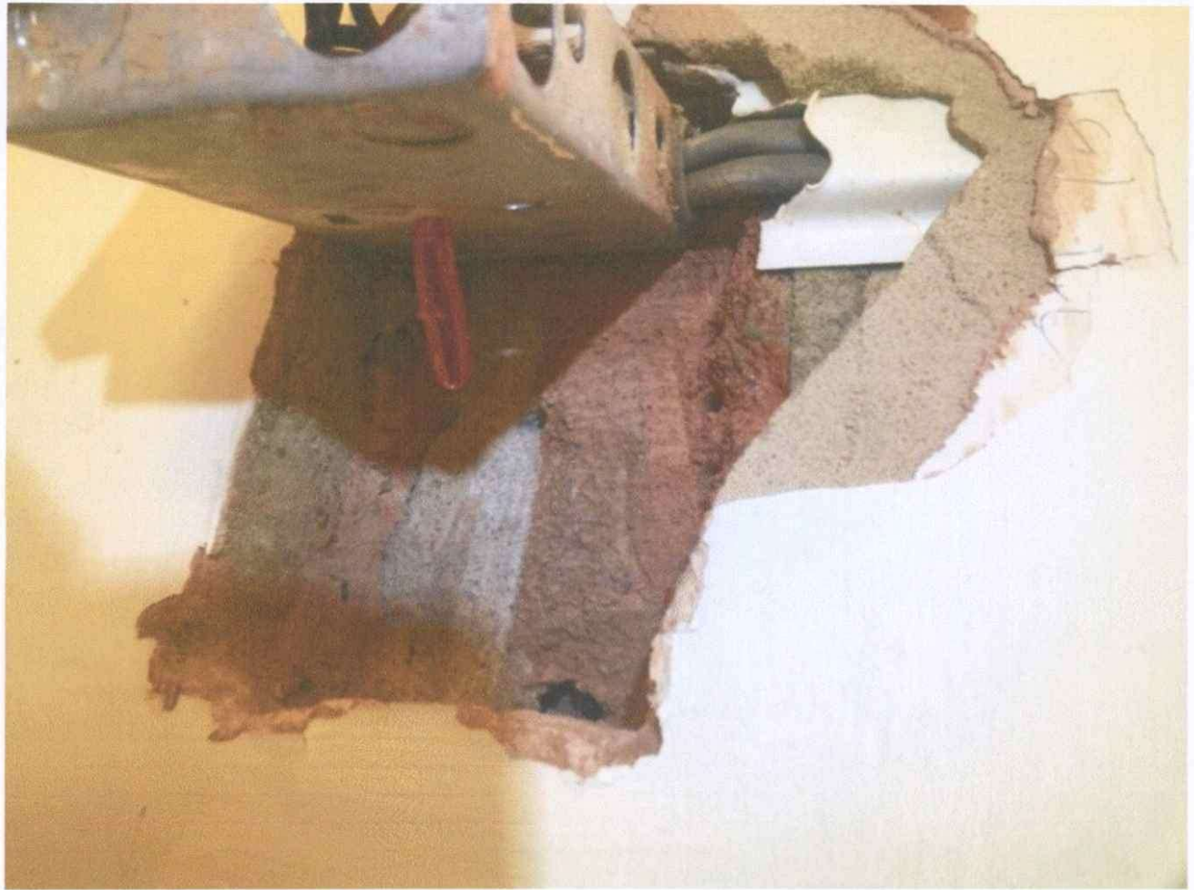
PHOTO 3 BRICK CONSTRUCTION INTERIUM KITCHEN WALL
