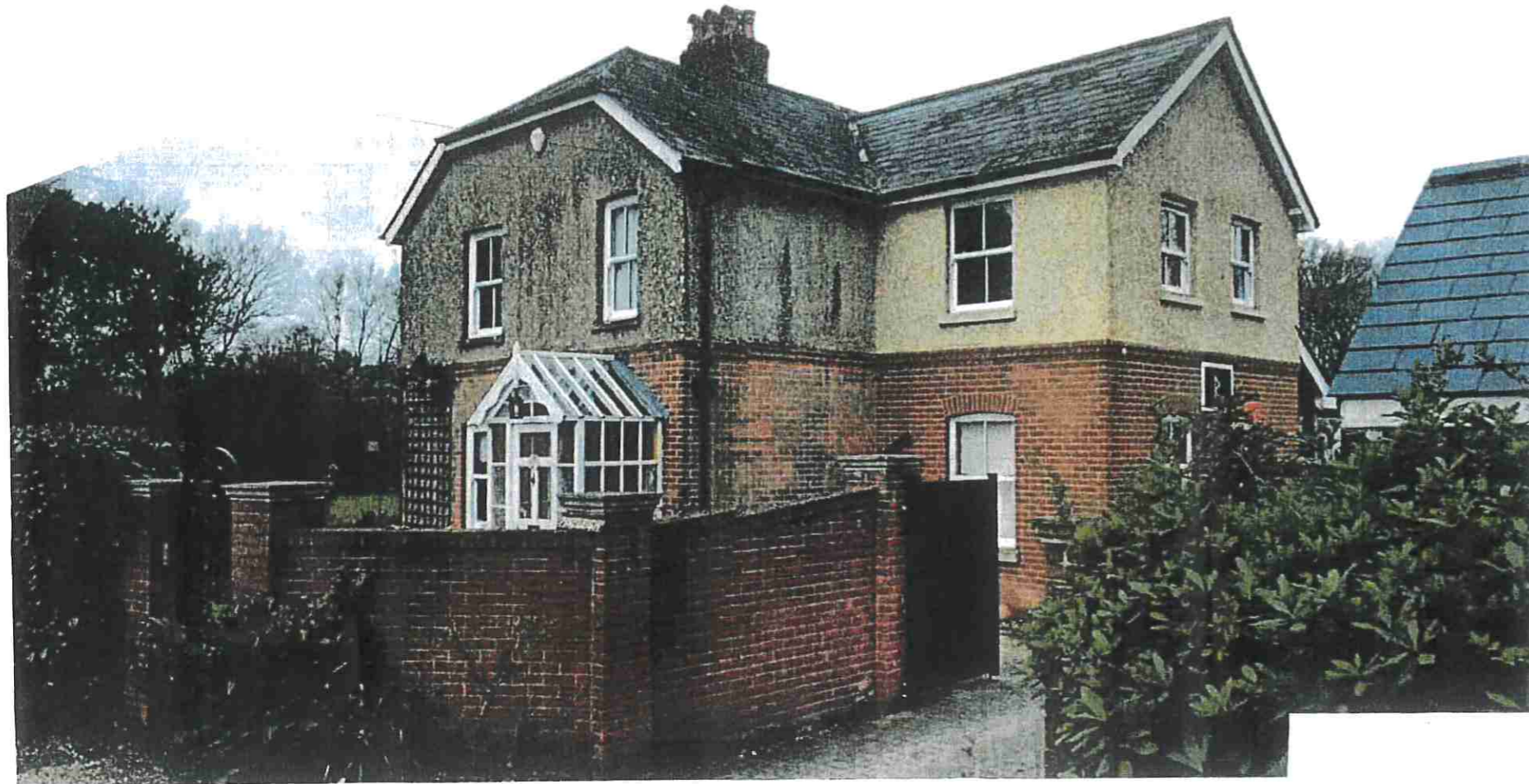
PHOTO FROM ROCKBOURNE ROAD, EXISTING PORCH.
