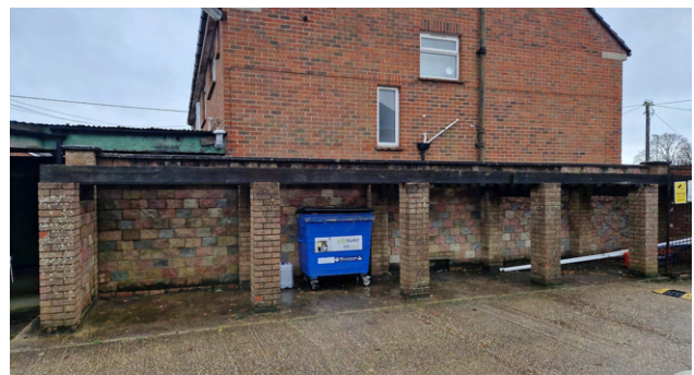
Refuse store area as existing
