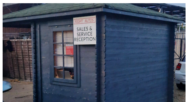
Existing Sales Office building
